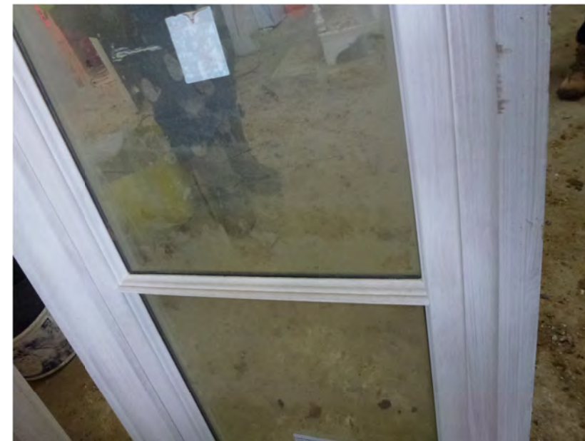
Sample proposed window mock-up by contractor. Glazing bar detail.
