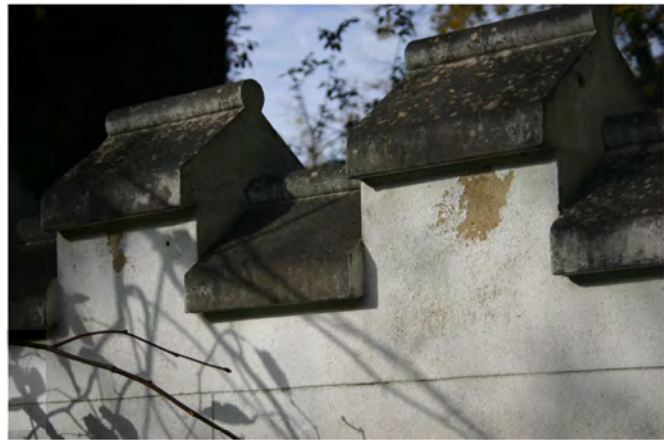
Existing castellated stone coping parapet detail to existing garage.
