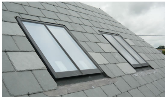
Example of conservation rooflights
