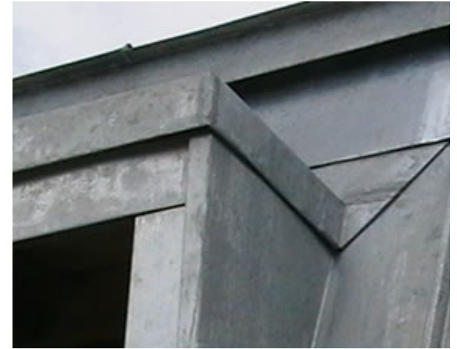
Example of zinc clad dormer
