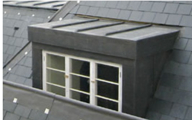
Example of zinc clad dormer
