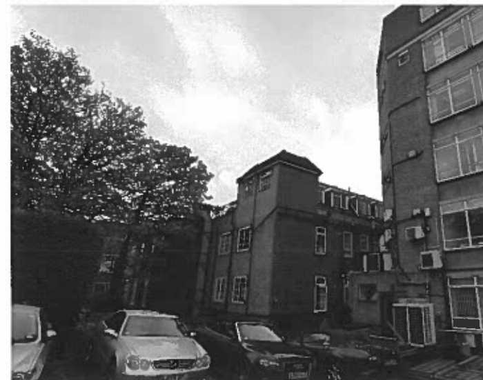
10 Rear of office building
