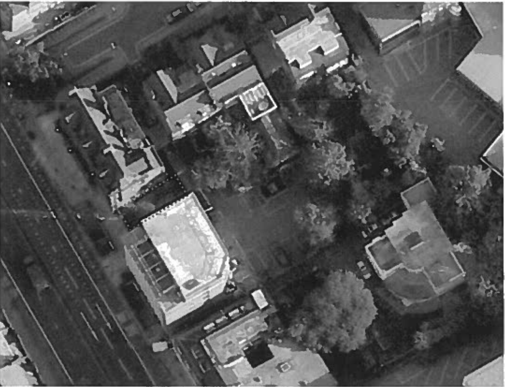
03 Aerial view of the site
