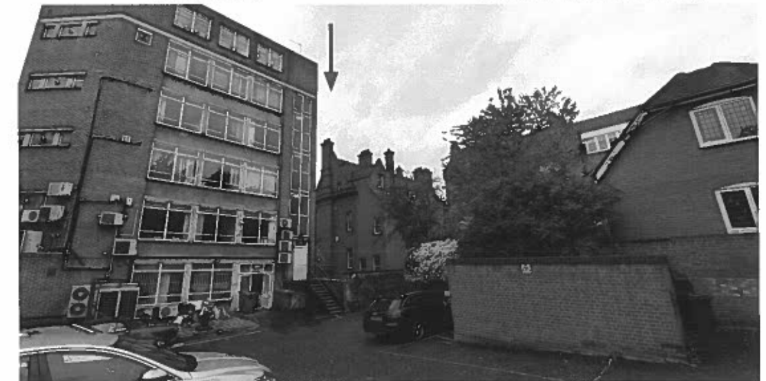
10 Rear view of site
