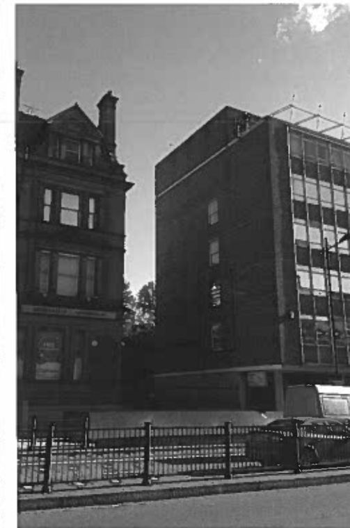
05 Flank wall - Office building
