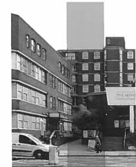
F - Gap 120 Finchley Road & Church
