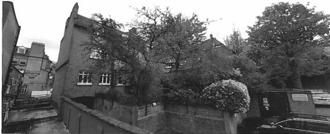
01 Rear of site, access road and neighbouring gardens opposite
