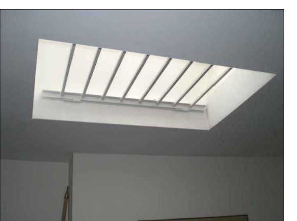
PHOTOGRAPHS SHOWING EXISTING SKYLIGHT AND THE ZINC ROOF
