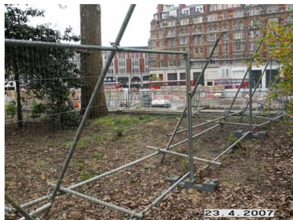
Effective fencing in position
