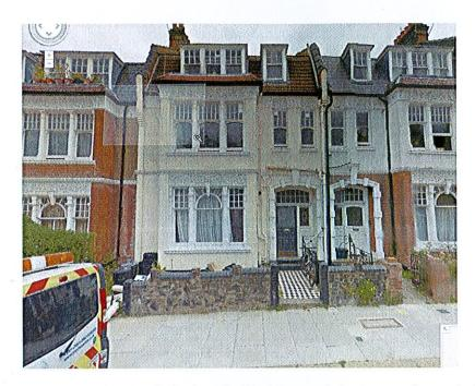
It comprises a tiled, mansard type pitched roof with dormer windows over the main house, timber suspended floors and painted brickwork walls. The rear addition comprises a tiled, mono-pitched roof.
