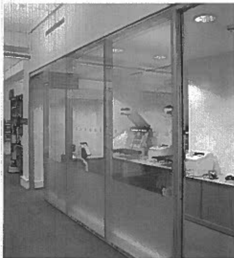
Existing glazing systems for reuse - Faram P500 @ Second Floor
