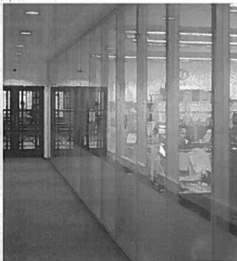
Existing glazing systems for reuse - Faram P500 @ Third Floor
