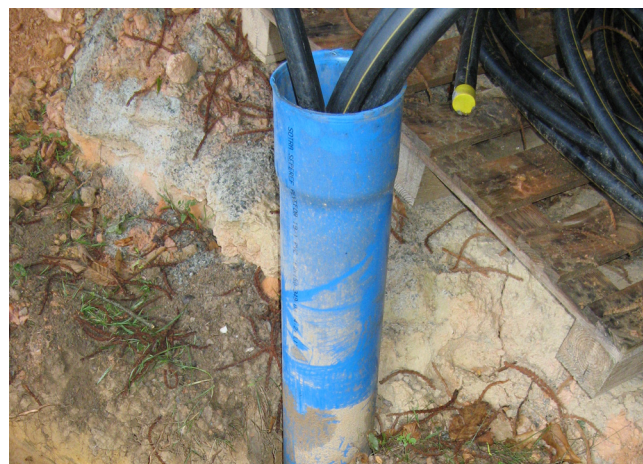
Example of GSHP borehole pipework.
