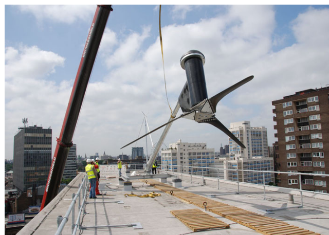
A building-mounted 6kW Proven wind turbine
