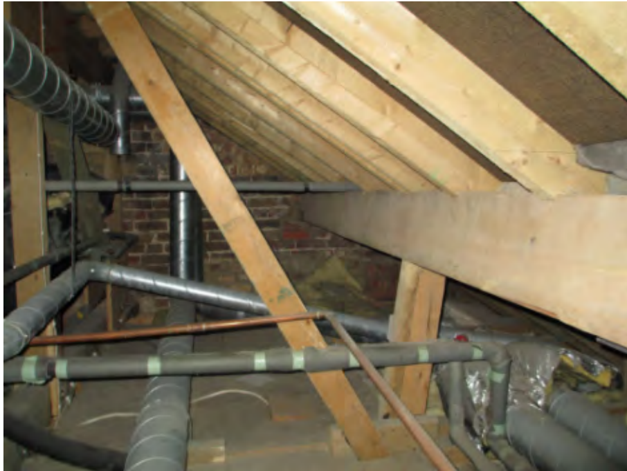
Photo 15 – Timber roof rafters and purlin, party wall behind
