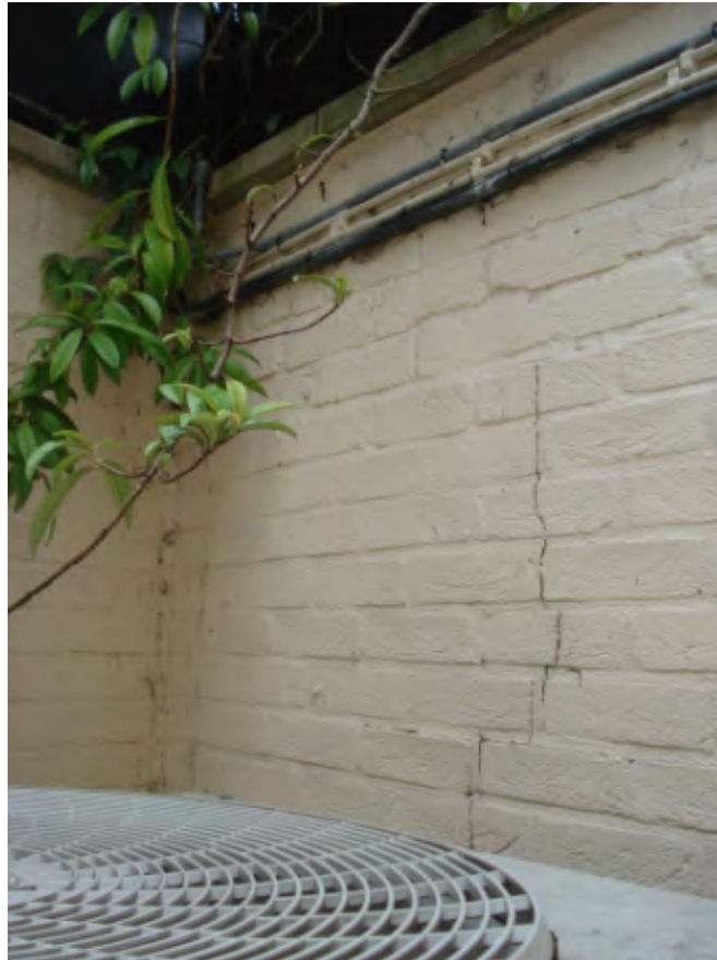
Photo 35 – Cracking to chiller compound wall
