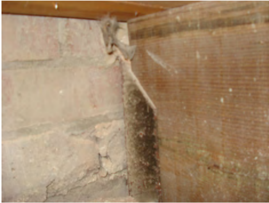
Photo 27 – Metal joist hanger (1960's)
