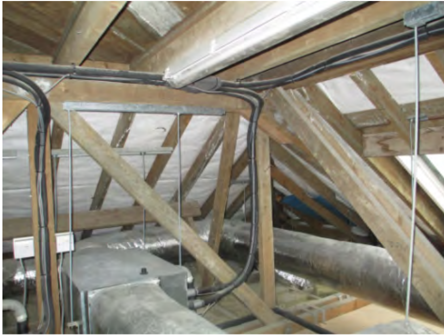
Photo 21 – No. 41 Roof corner – primary and secondary trusses
