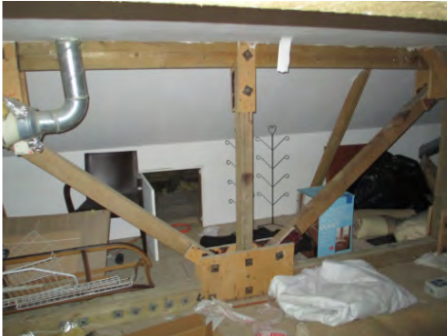
Photo 11 – No. 42 Roof primary truss
