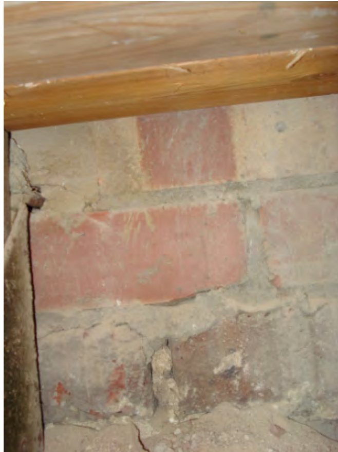
Photo 29 – Fletton brick repair (1960's)
