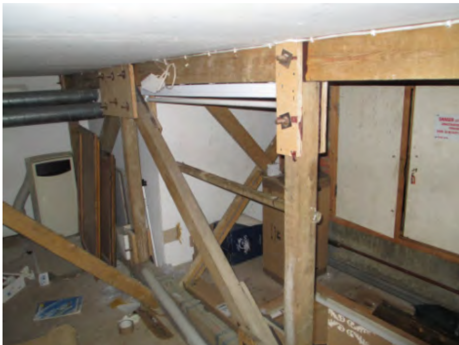
Photo 12 – No. 42 Roof primary truss
