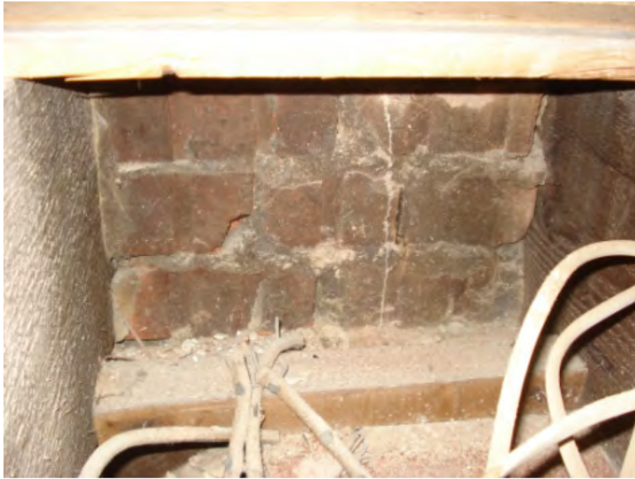
Photo 31 – Fletton brickwork to stair enclosure (1960's)
