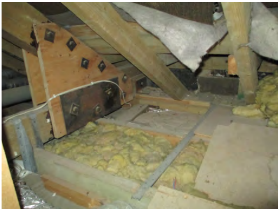
Photo 18 – No. 42 Roof main truss bottom connection
