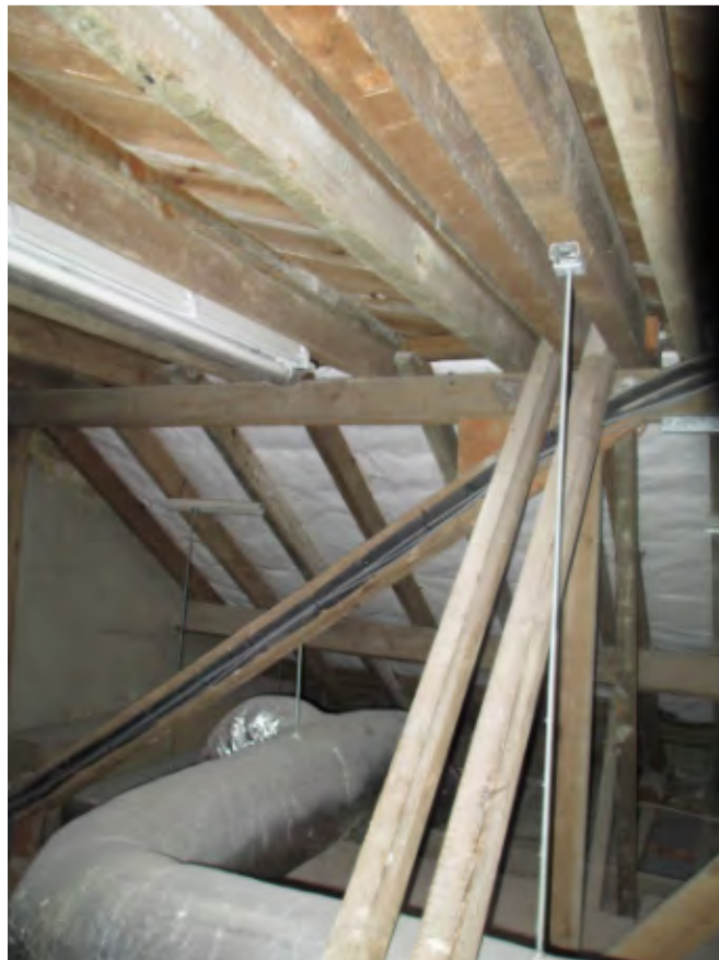
Photo 26 – No. 41 Timber joists supported on primary truss
