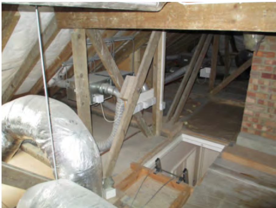
Photo 24 – No. 41 Secondary truss and loft access hatch
