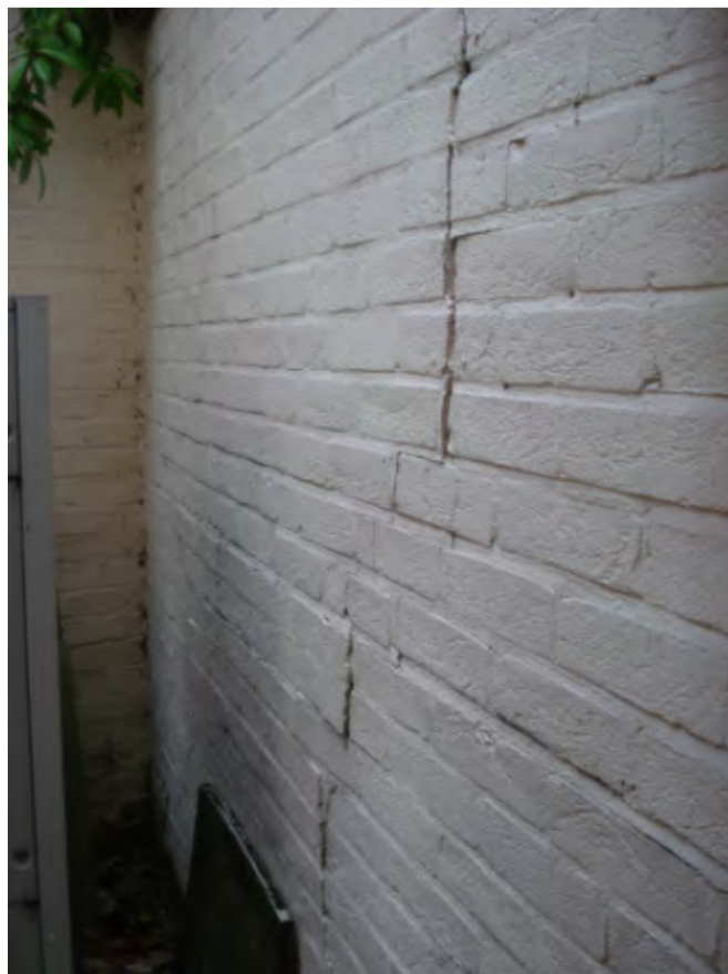
Photo 36 – Bulge and cracking of chiller compound wall
