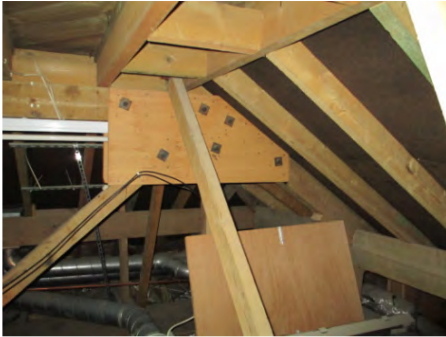
Photo 17 – No. 42 Roof main truss top connection
