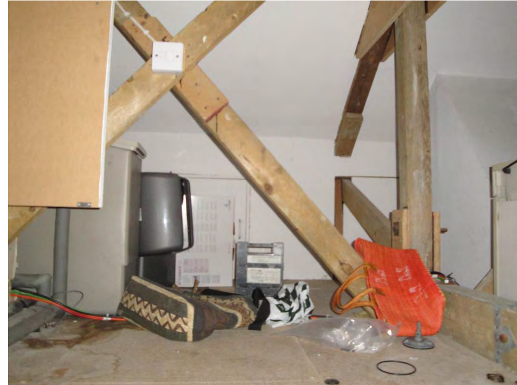
Roof area – evidence of earlier strengthening works
