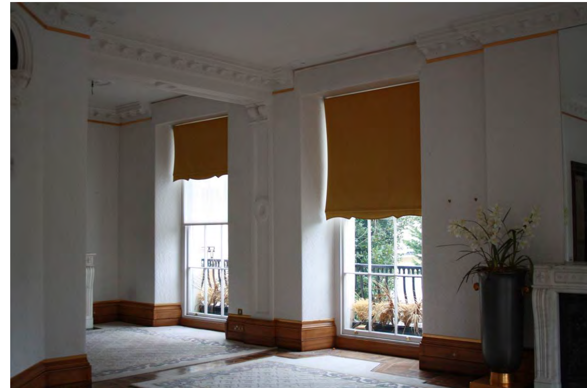
Modern skirting - behind concealed electrical and mechanical installations
