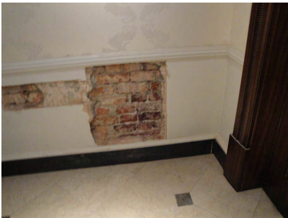
Investigative opening – Ground floor – entrance area party wall– fletton brick infill; cement rendering
