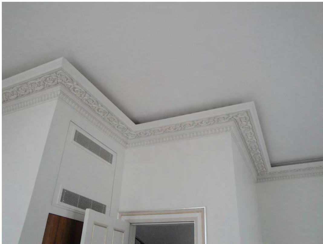
First floor Living Room - - air condiitoning vents; modern cornice, with shadow gap
