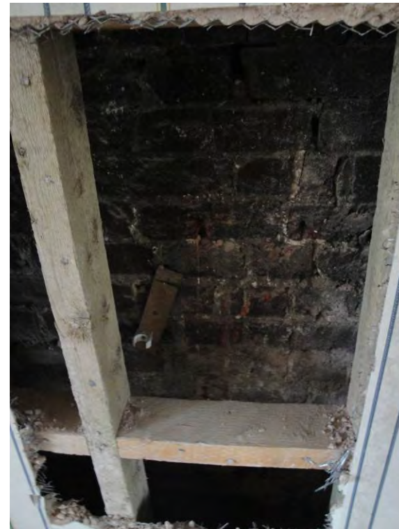
Wall – boxing to create space for installations, affects plan form
