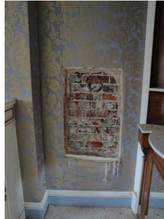
Third Floor Opening in party wall - cement render over modern Flatton bricks
