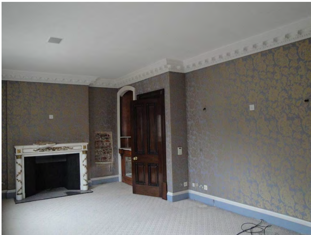
Elaborate fireplace- not original; Walls covered with decorative fabric; elaborate modern joinery, later; modern cornice, skirting, ceiling with services fittings.
