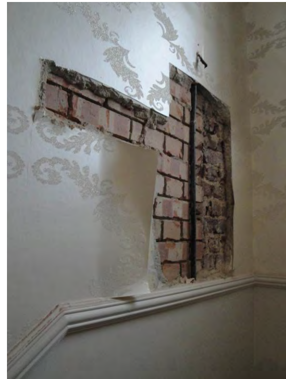
Investigative opening – party wall - landing reveals more infills – Fletton bricks
