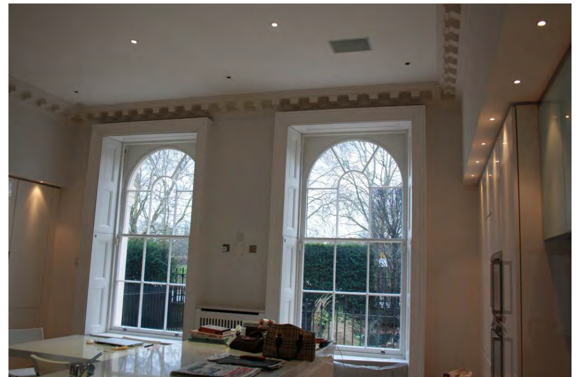
Ground floor – view towards Regents park The cornice, ceiling and joinery are all new, note recessed downlighters and services in ceiling, boxed out soffits.
