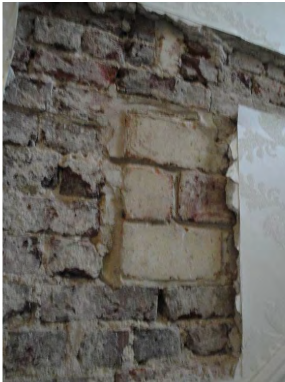
Investigative opening – party wall - landing reveals more infills – Fletton bricks
