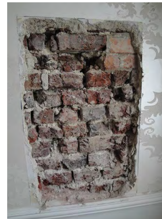
Opening on the First Floor Landing – party wall, more infills revealed – cement render damage to the brickwork
