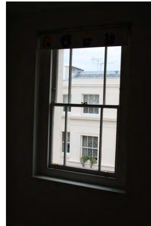
3-o3 sash window, later joinery and ironmongery
