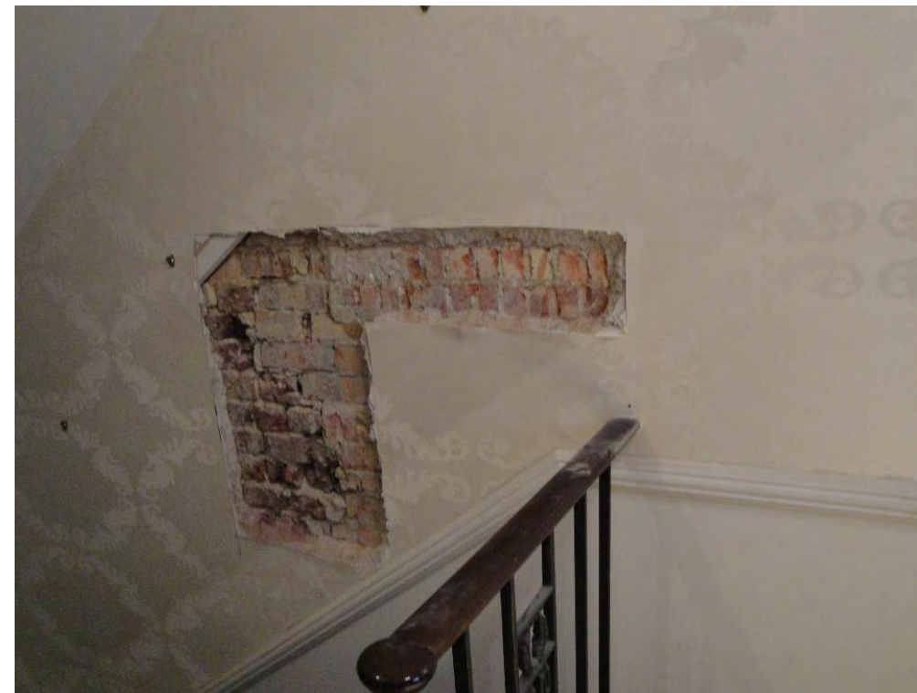
Investigative openings, revealing fletton bricks infill in the party wall
