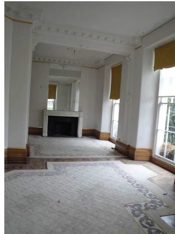
Room layout changed - partition wall between two rooms removed, creating awkward narrow layout
