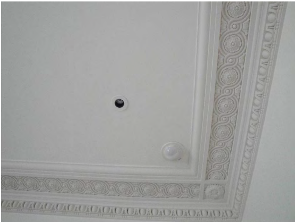
Third floor - ceiling in bedroom; elaborate cornice, inappropriate size for this floor, services
