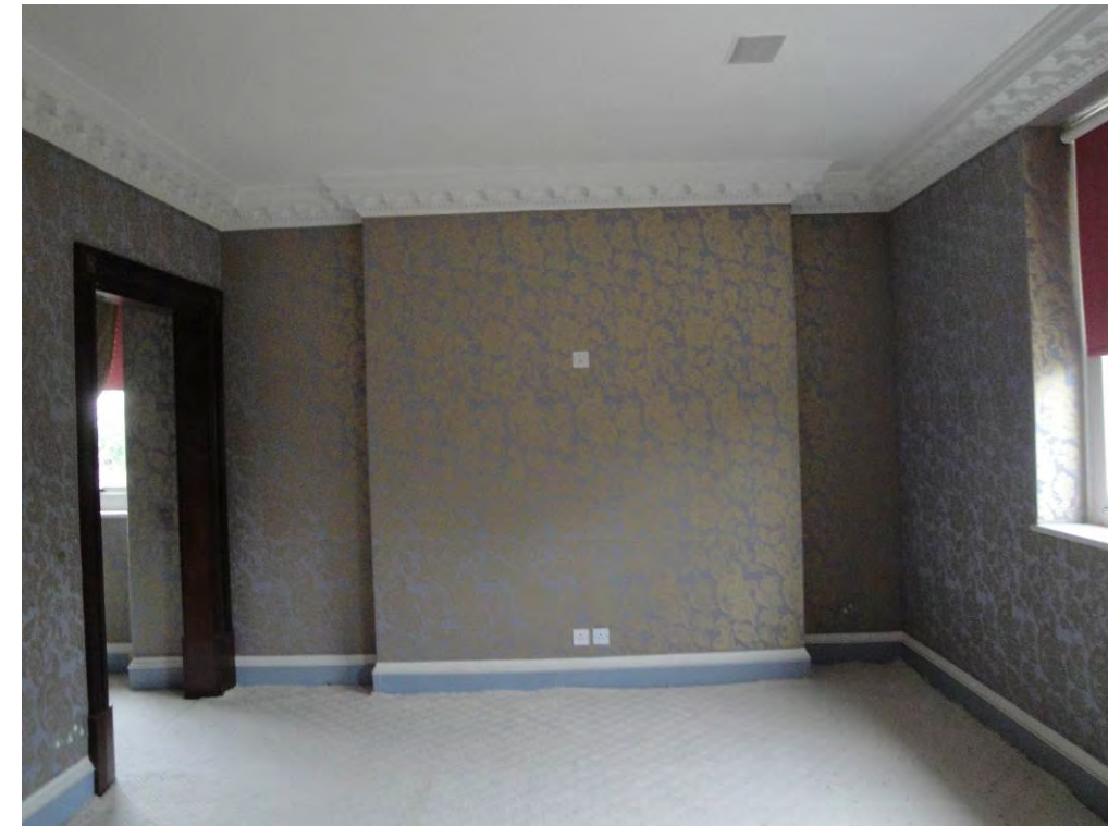
Fireplace missing – all modern joinery plasterwork and floor structure.
