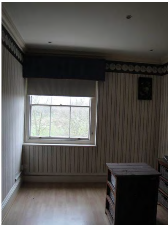
Bedroom - partition wall close to window, later modern cornices; ceiling plaster, downlighters;
