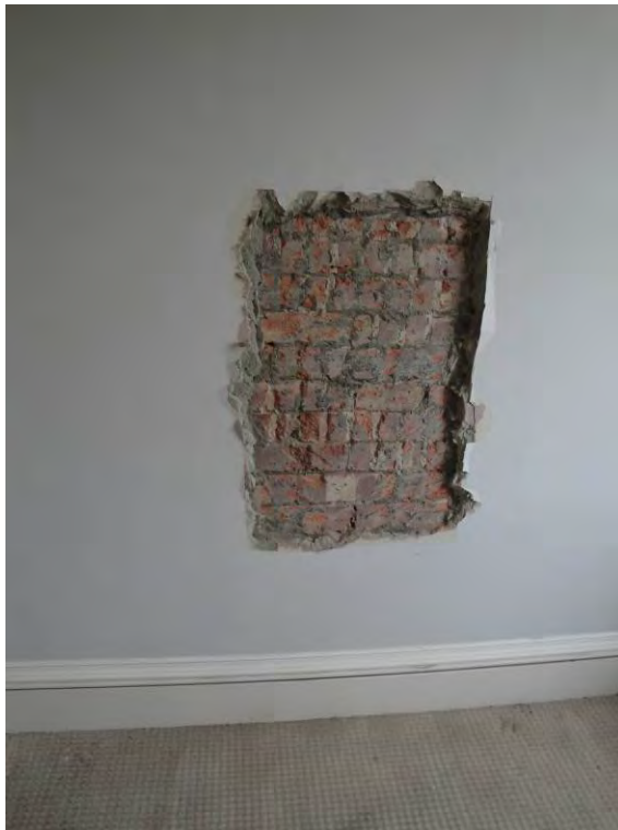
Opening to party wall reveals modern construction
