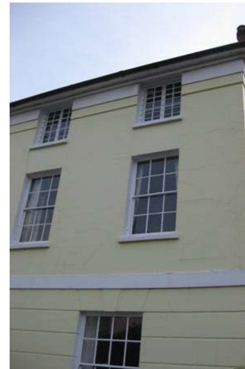
1.6 Rustication at upper ground floor level
