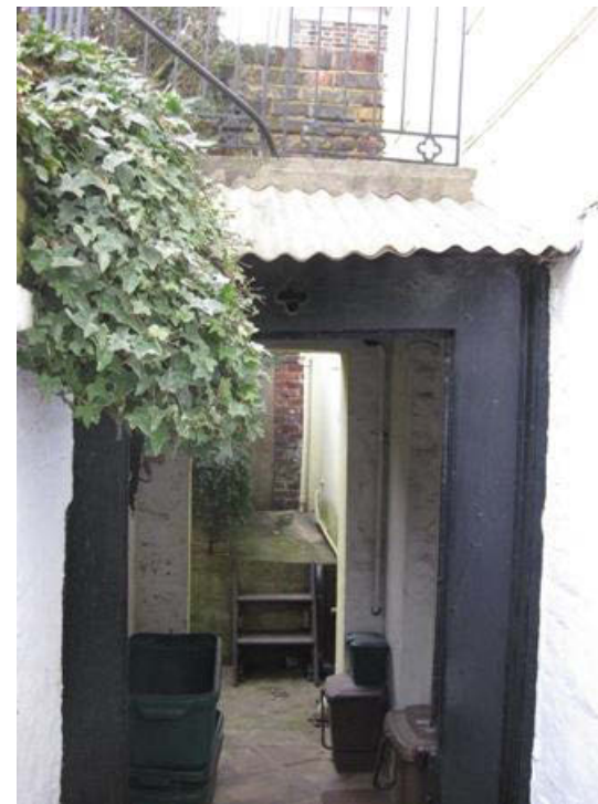
1.12 "Lean-to" structure next to the entrance bridge
