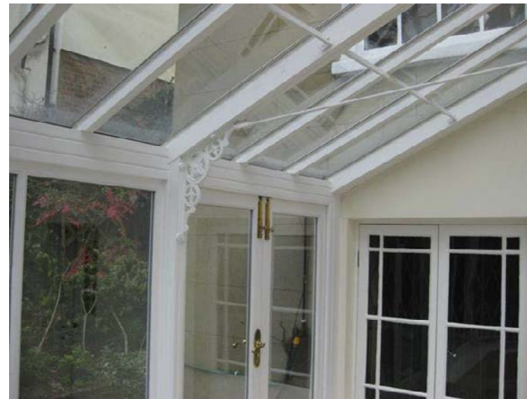
3.26 Doors to dining room
