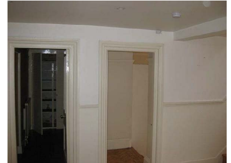
3.3 Doorways between kitchen and 1925 wing
