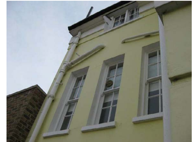
1.3 Front elevation of 1925 wing
