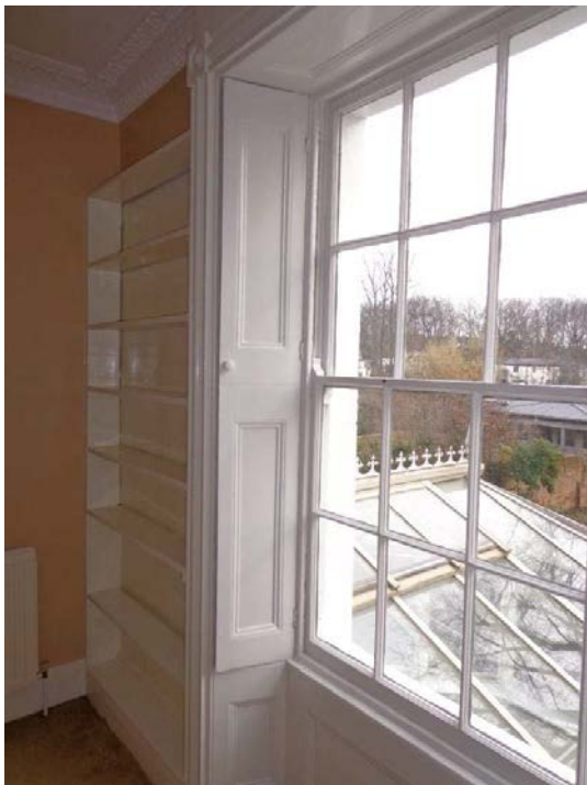
3.38 Timber sash window and shutters
