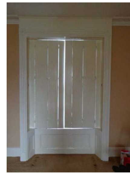
3.36 Timber sash window with shutters
