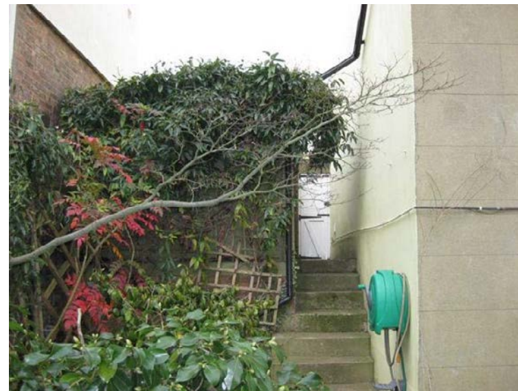
1.19 Rear of garage
