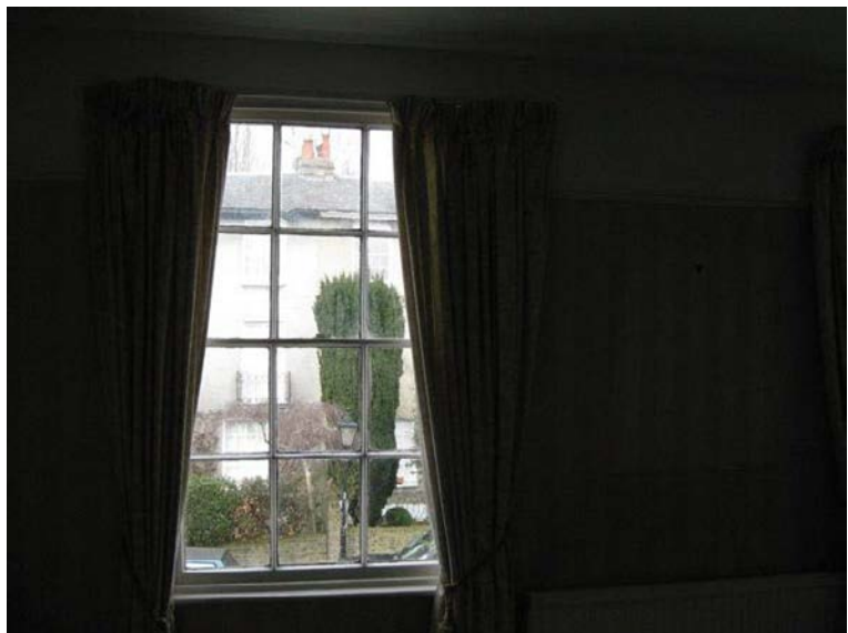
3.73 Timber sash window
