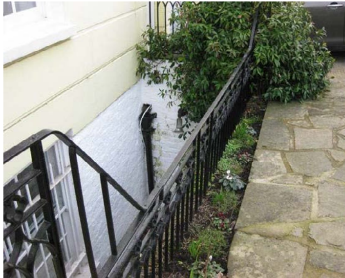
1.8 Railings and lightwell
