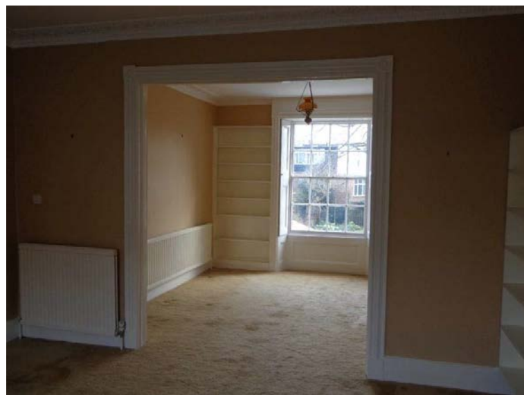
3.34 Opening between UG1 and UG2
