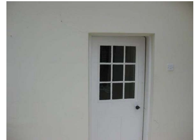
3.27 Doors to corridor/stairs
