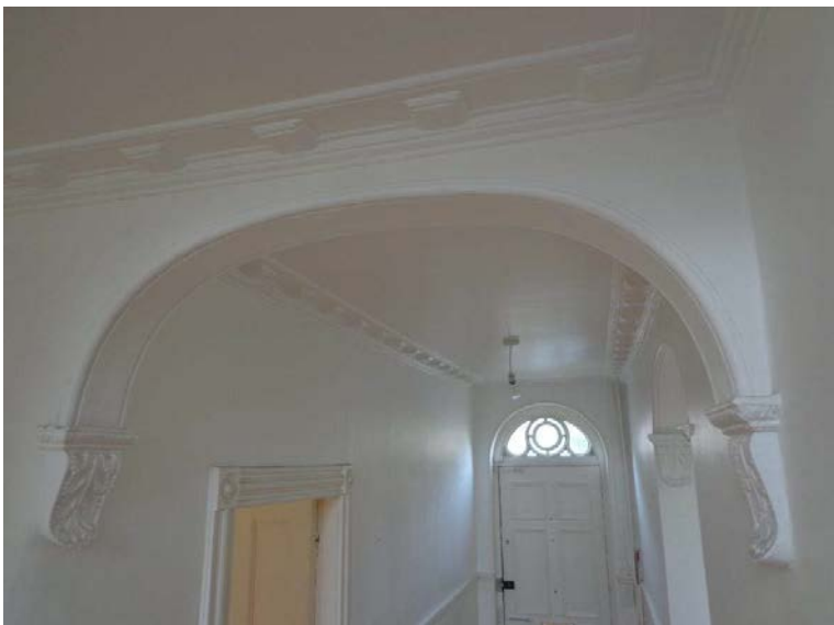
3.47 Arch with mouldings
