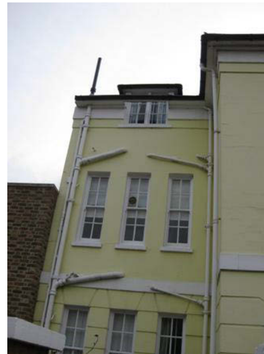
1.5 Front elevation of 1925 wing
