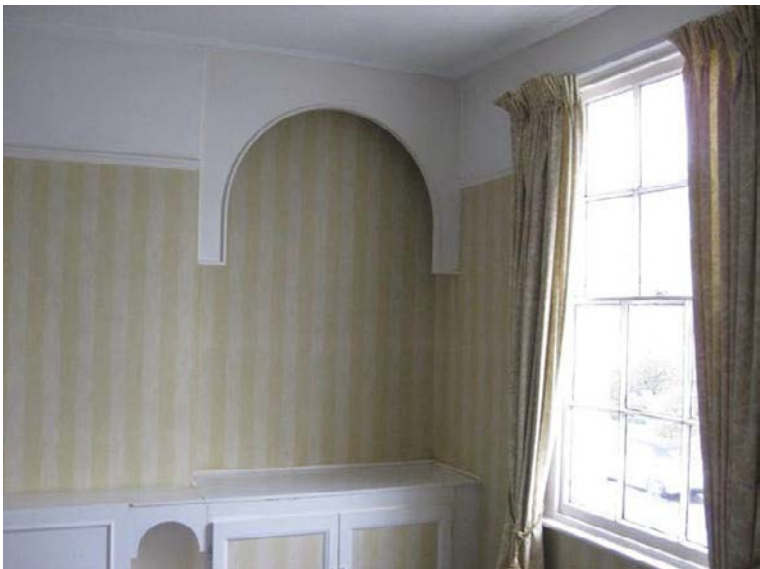
3.72 Timber sash window
