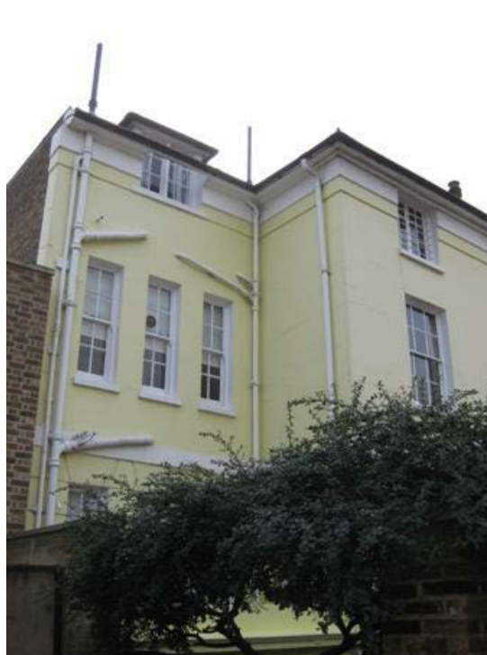
1.4 Front elevation of 1925 wing
