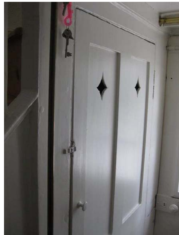
3.17 Door to under-stair area
