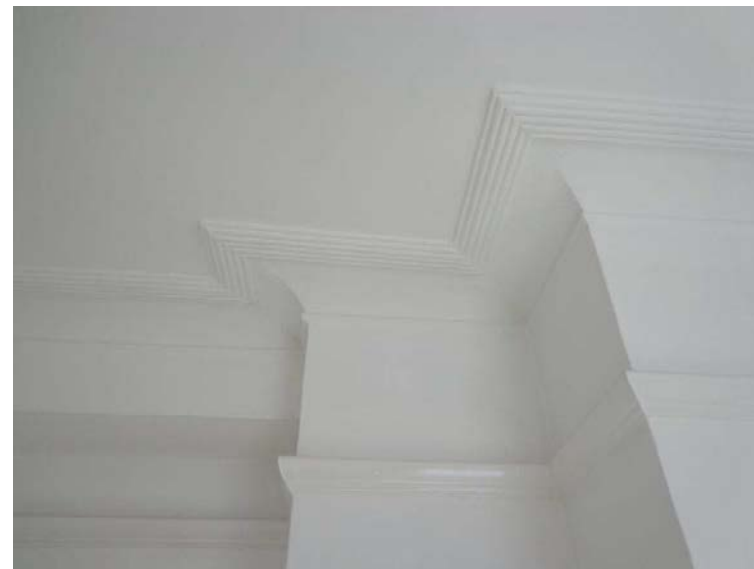
3.61 Typical 1920s detailing
