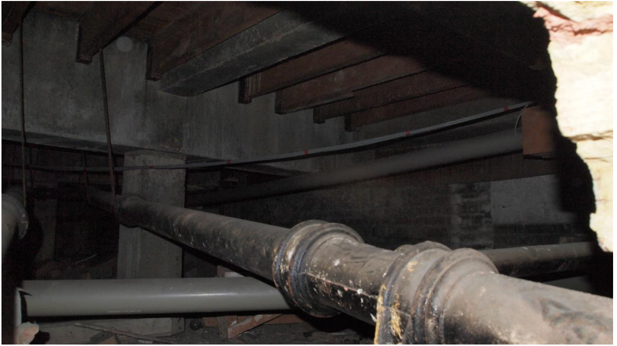
Suspended ground floor structure to rear of existing property (area of new basement)
