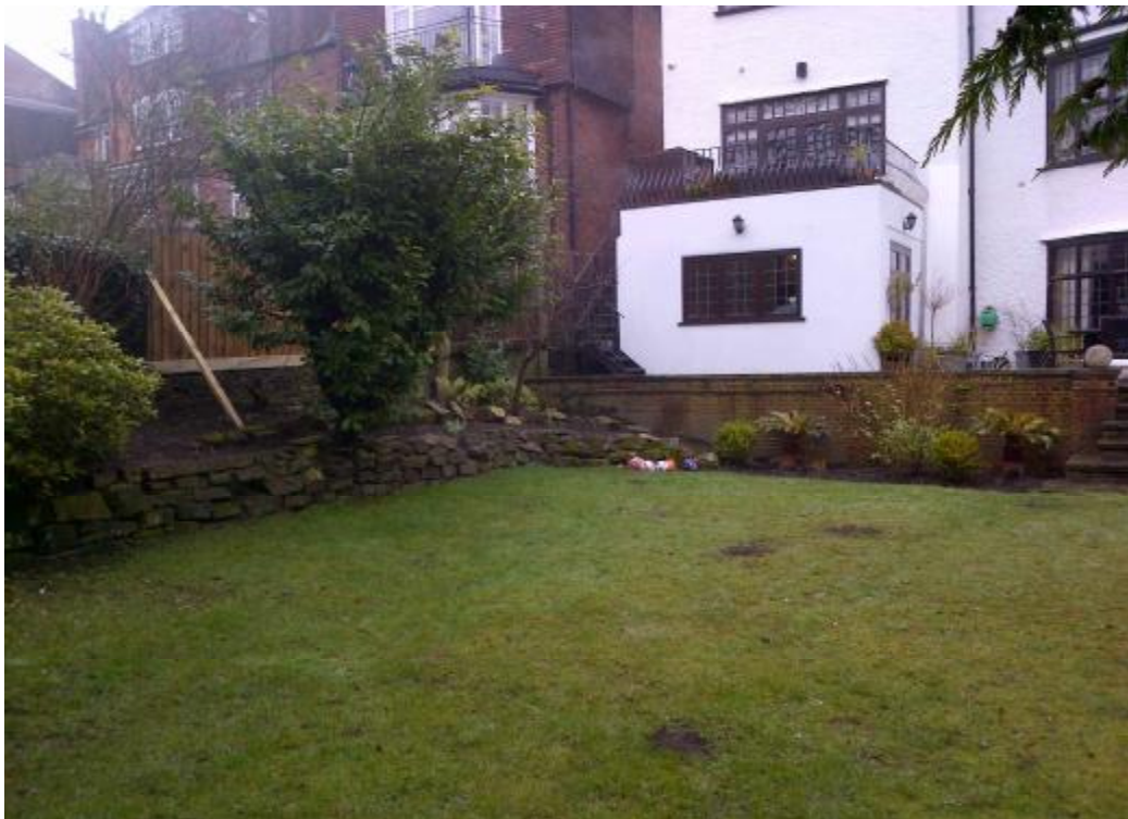
Photo 2: Northern side of rear garden, where proposed basement will extend out beneath the lawn. Note retaining walls below boundary fence and supporting terrace, and dry stone wall to flower bed.
