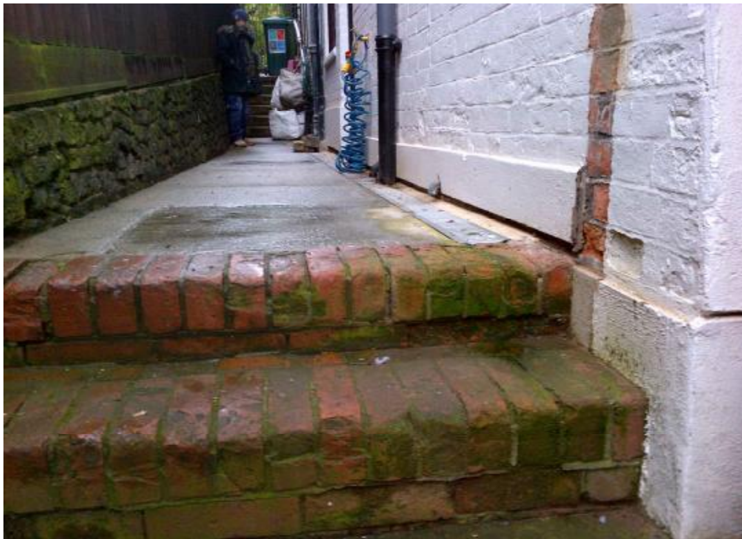
Photo 11: Path alongside north flank wall, showing settlement relative to wall and new drain.
