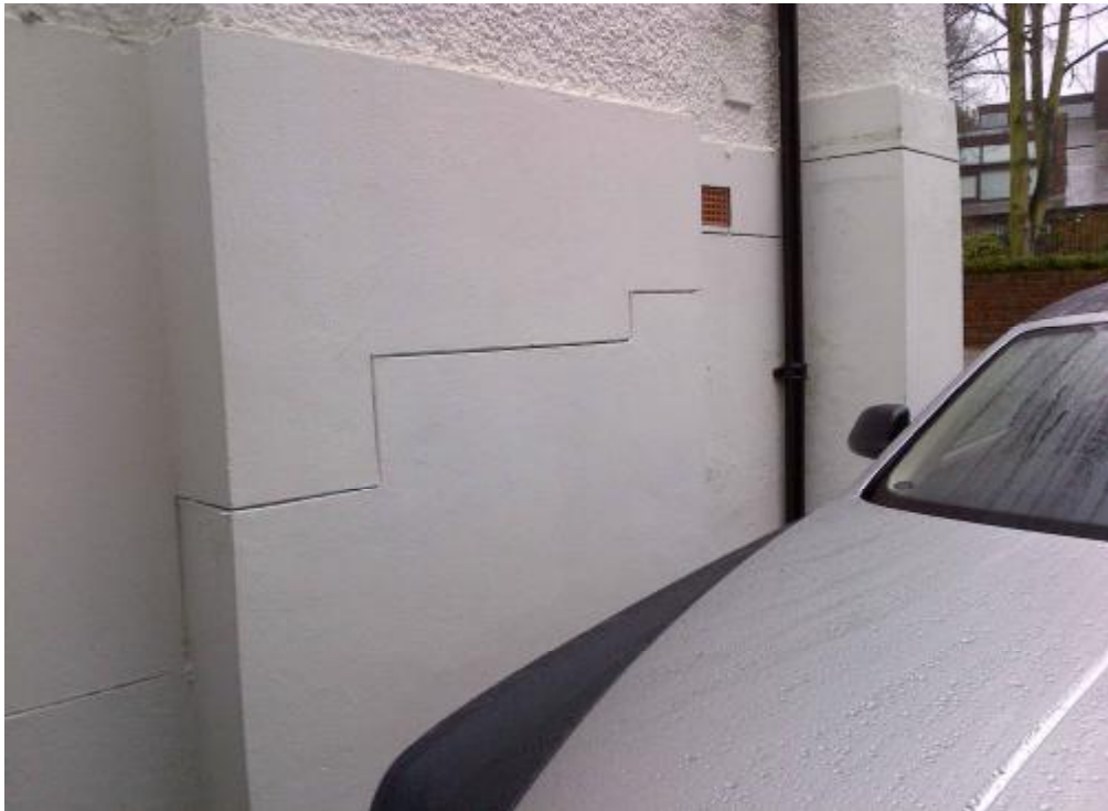
Photo 12: Stepped groove in render which probably marks position of damp proof course, with wall below that level retaining the inclined earth as seen in the crawl space beneath front part of house.
