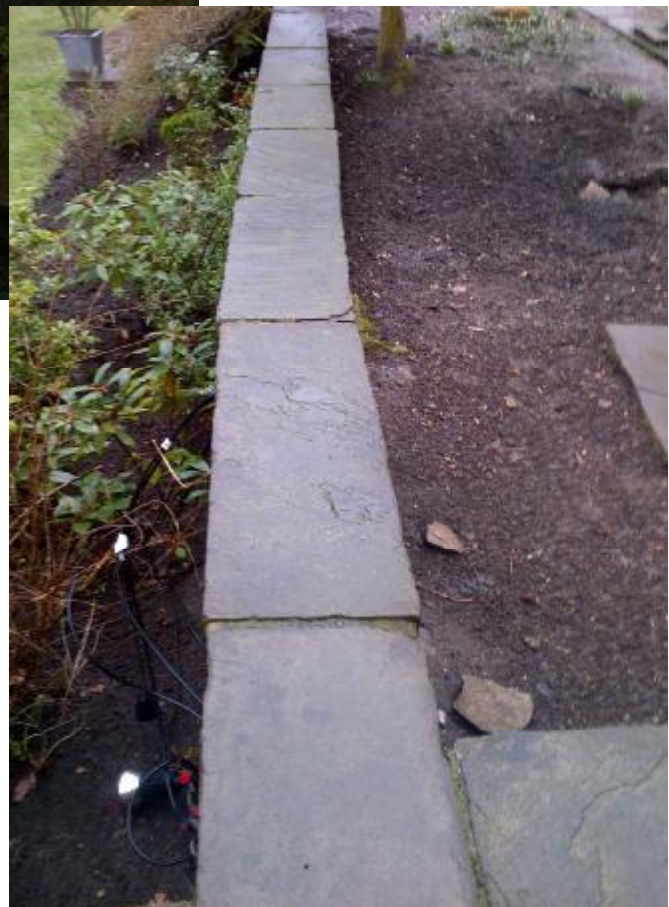
Photo 9: South end of retaining wall supporting terrace, showing outward displacement.
