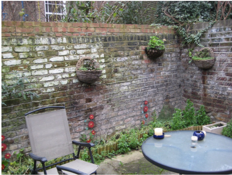
View of rear elevation
