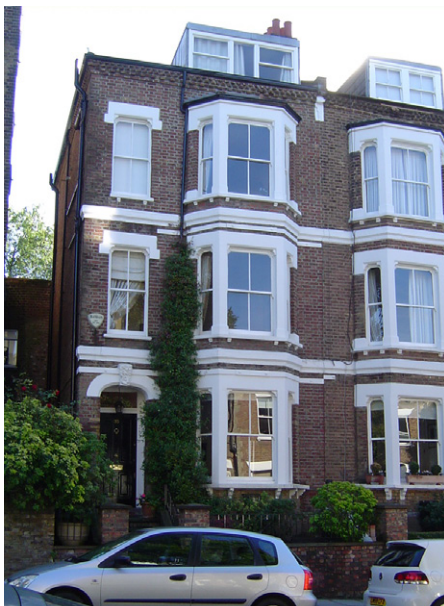
view of front facade
