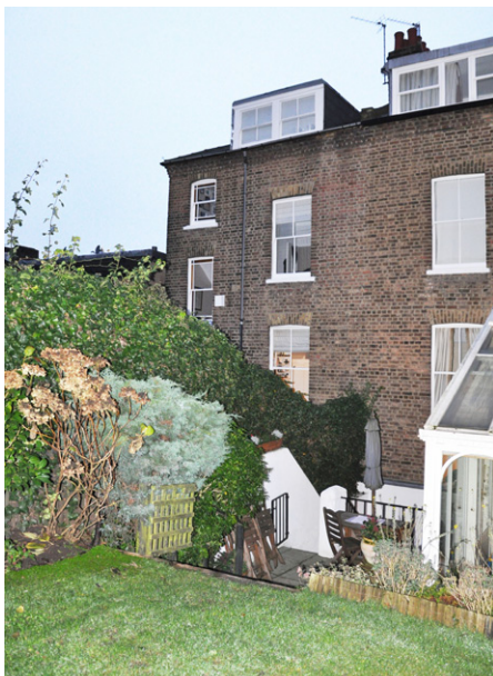
view towards boundary with no. 33
