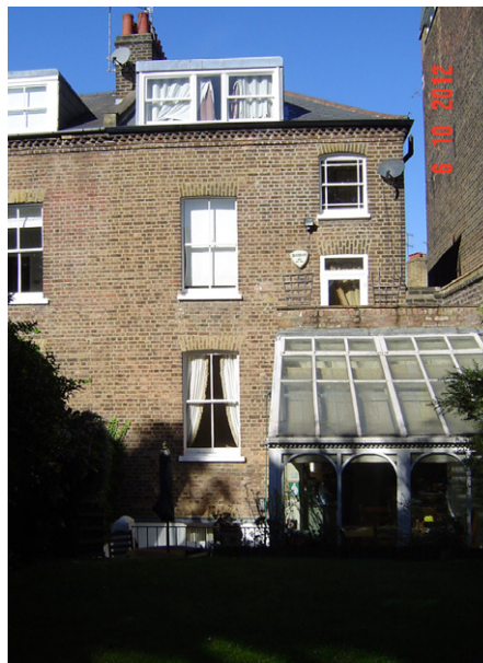
view of rear facade
