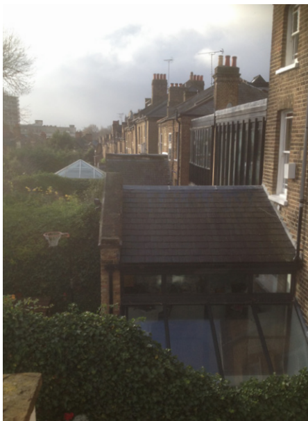
current overlooking issues from second storey roof terrace to be addressed and significantly improved
