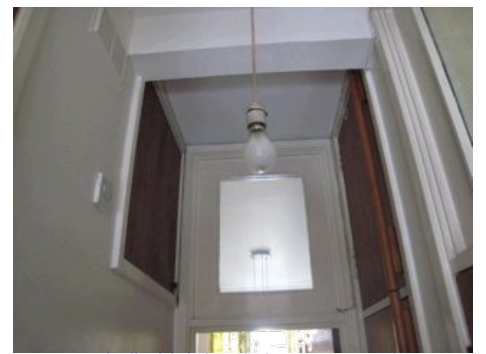
entrance hall - high level view
