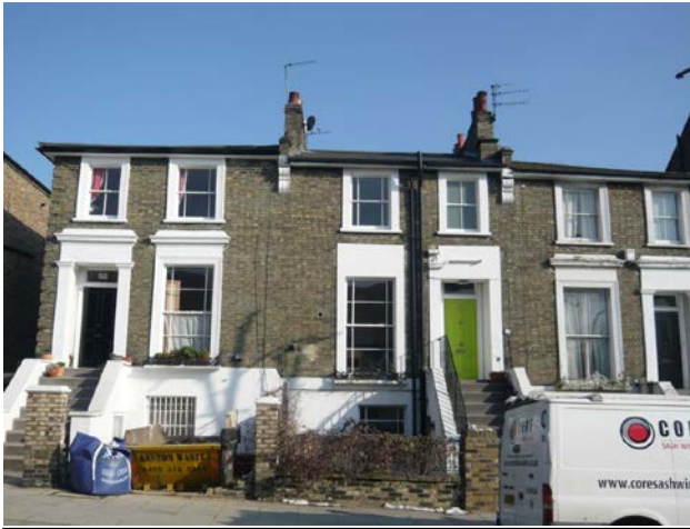
Existing front view
