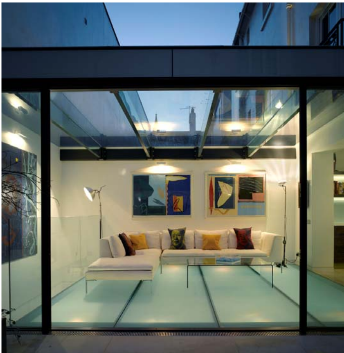
Fig 4 – No. 5 Park Village West, view of similar extension, with powder coated steel frame and sliding glass doors
