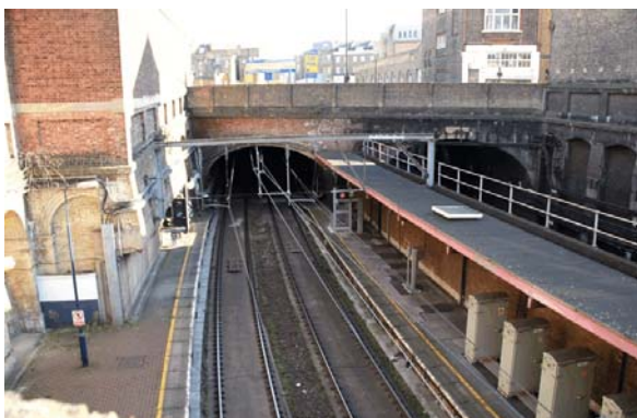
Thameslink Tunnel Opening Under Site
