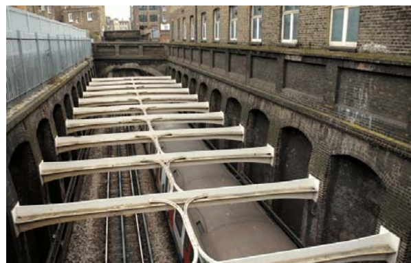
Circle Line Train in Cutting: site railings to the left
