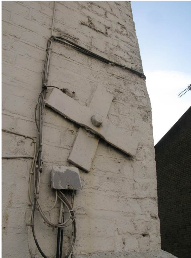
PHOTOGRAPH 1 Tie bar end, North West end
