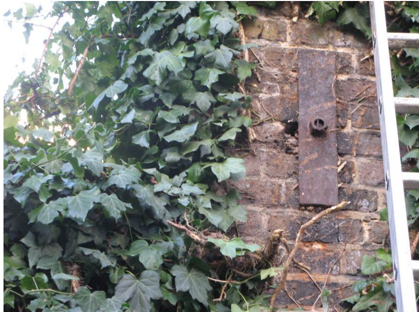
PHOTOGRAPH 2 Tie bar end, South East end
