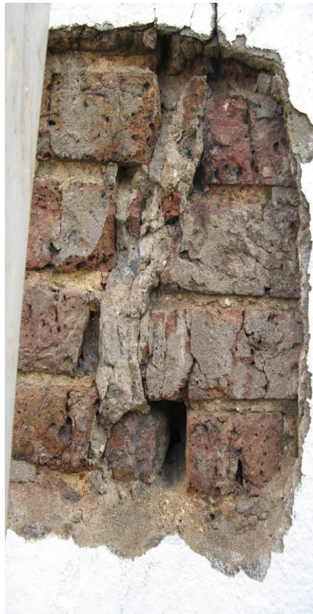
PHOTOGRAPH 4 Masonry fracturing
