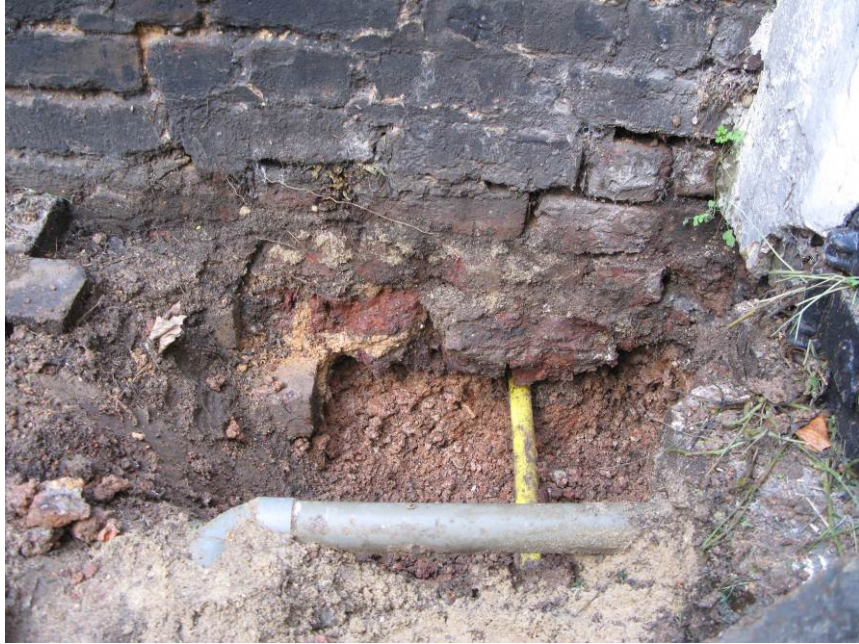
PHOTOGRAPH 3 Dilapidated brickwork
