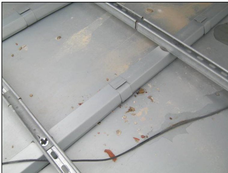
Fig 2 Attachment of solar panel frame to uprights of zinc roof
