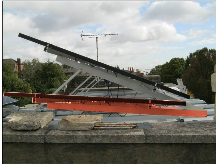
Fig 3 West elevation view (ie looking east) of panels and mounting frame. The nearest panel is that visible from the public realm. The red 'panel' indicates the position to which the panels will be lowered.
