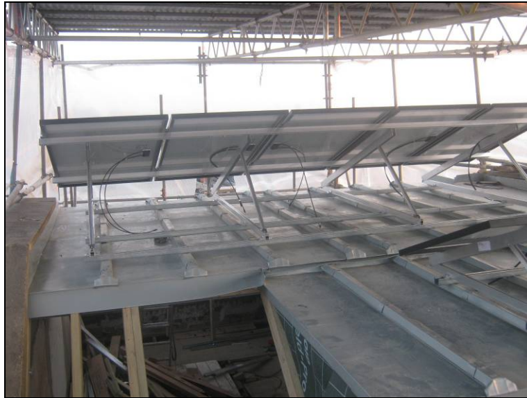
Fig 1 Installation of solar panels during the roof restoration.
