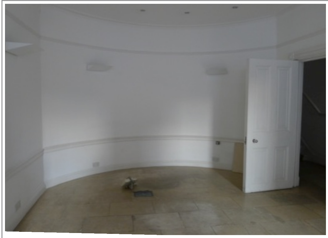
1. Curved wall to be demolished and rebuilt slightly further into the front room with a shallower curvature. The existing door will not be effected by the works.
