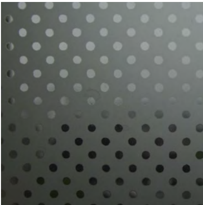
Existing reverse frit to WC areas & stair cores
