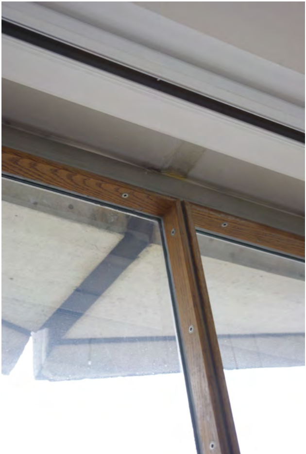
Photograph illustrating existing single glazing
