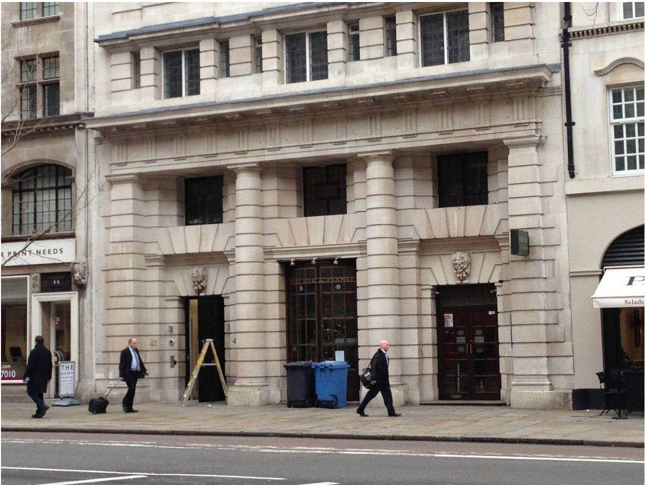
2. Part of Front Elevation – 42 Kingsway.
