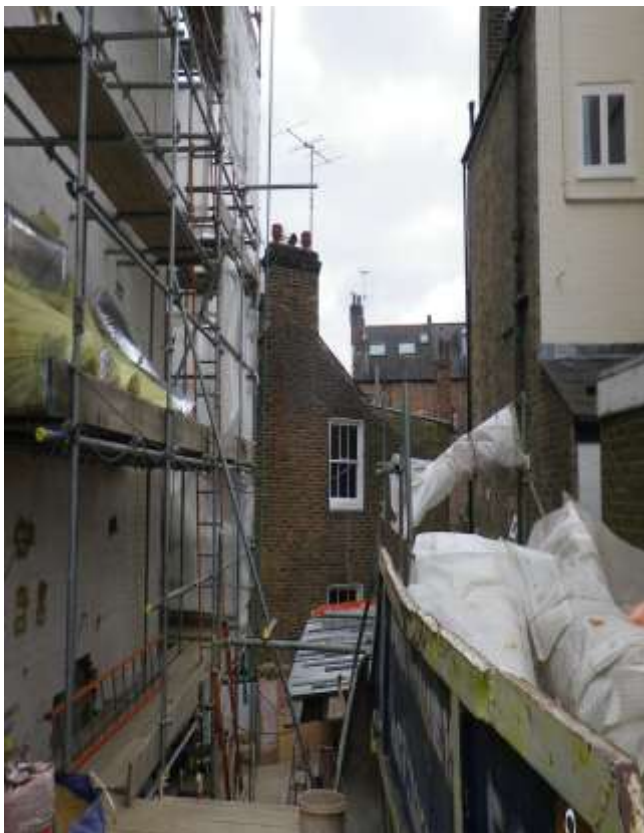
View south of windows at no.41 Willow Road
