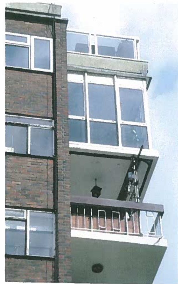
EXISTING BALCONY of FLAT no. 14
