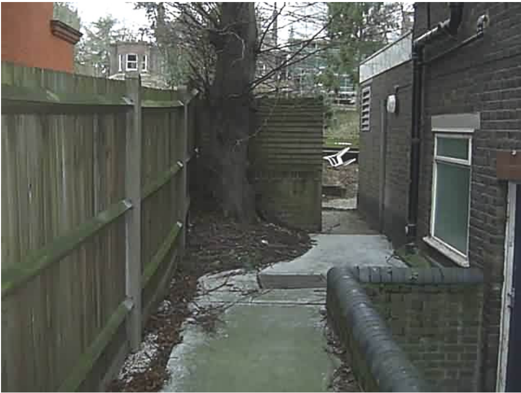
Built structures adjacent to Tree 2
