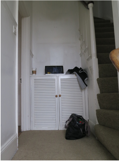
Second floor landing. Proposals to close existing opening and create opening straight ahead and to create access to understairs storage from landing. (REG/17-014)
