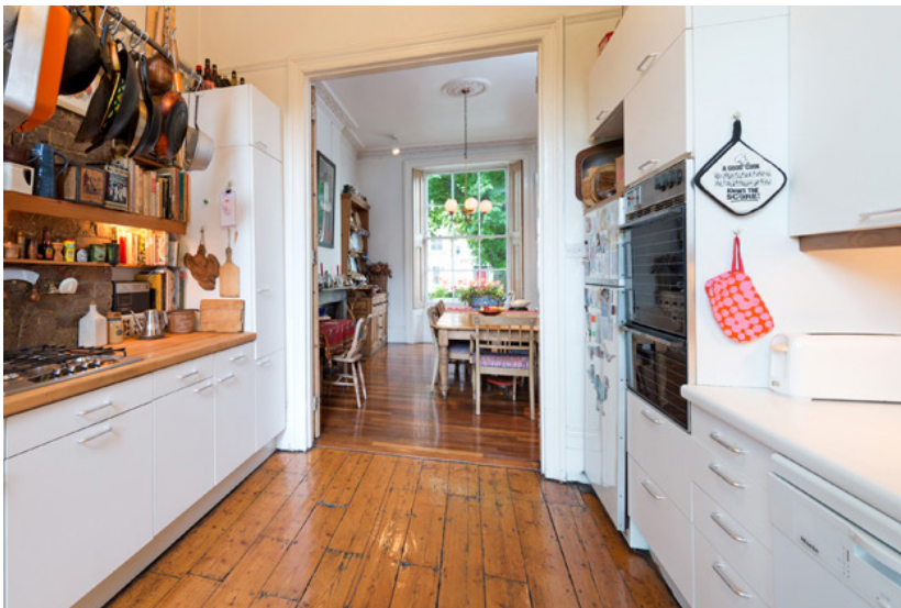
Existing kitchen to be removed and converted into dining room with sliding doors. Proposed opening on right side. (REG/17-012)
