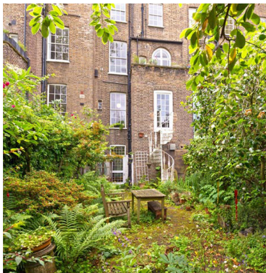
Rear elevation, addition of door on LGF behind stairs. (REG/17-019)
