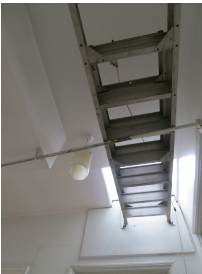
Internal view of existing roof light. (REG/17-015)
