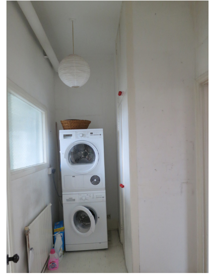
Existing utility room to be relocated to LGF and replaced with walk in closet. (REG/17-014)
