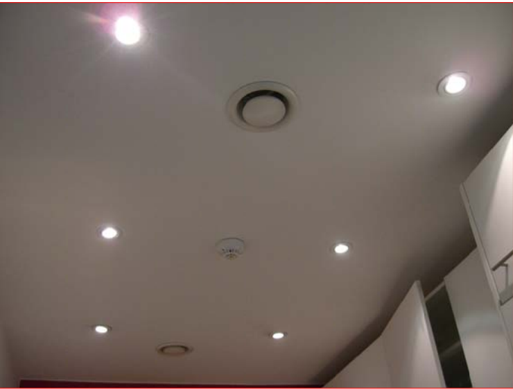
DOWN LIGHT (HALOGEN LAMP)
