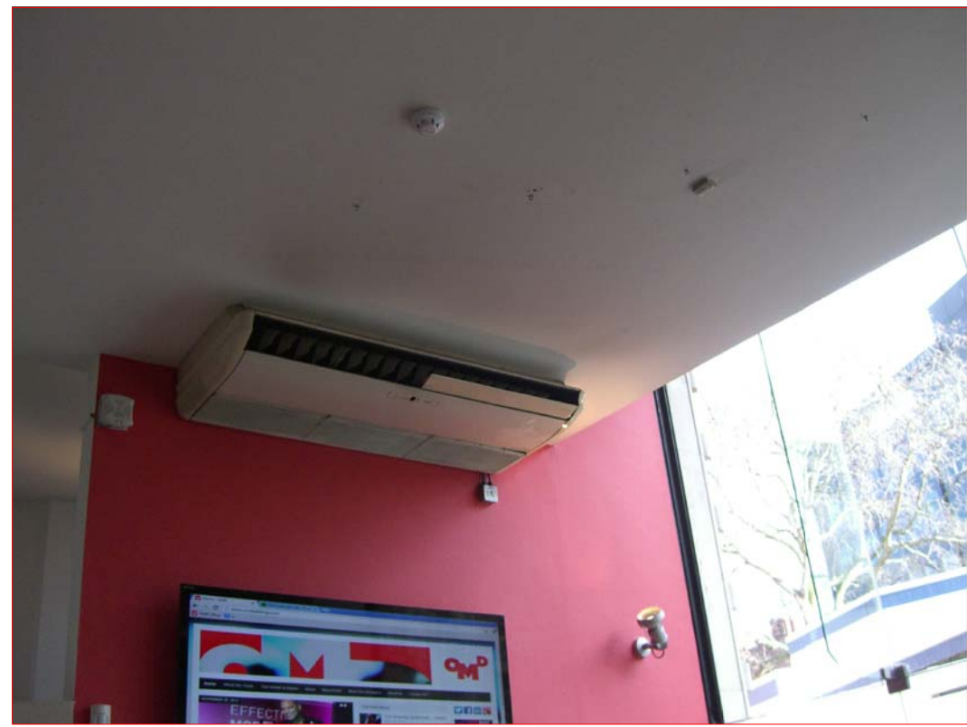
CEILING MOUNT TYPE A/C UNIT
