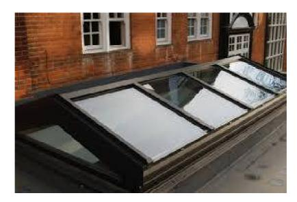
to an Em-Vault, polycarbonate in a dark grey powder coated aluminium frame as shown below:-
