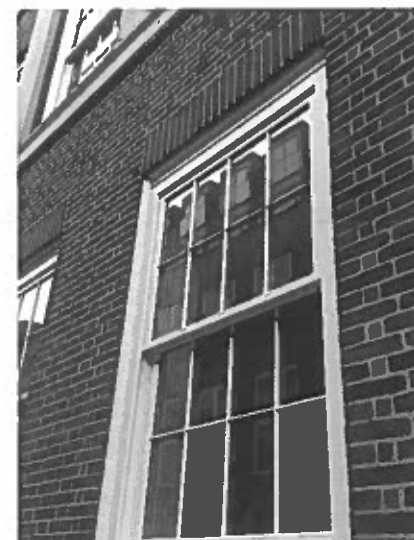
Fig.2 Precedent: Applied glazing bar with spacer at 3-4 Picton Place, London
