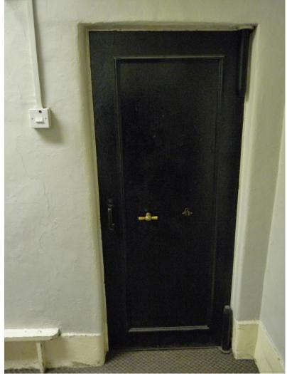
**APPENDIX I** Subdivided front ground floor room 24 with evidence of blocked up hatch.
