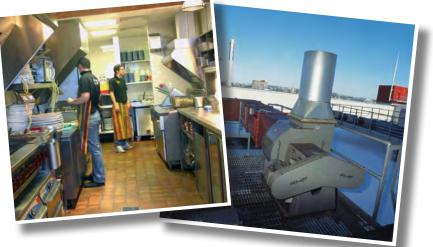
efficiency is heavily reduced. The UV-O range was designed with this in mind and as it is located outside of the air stream, pre-filtration is not a necessity.
