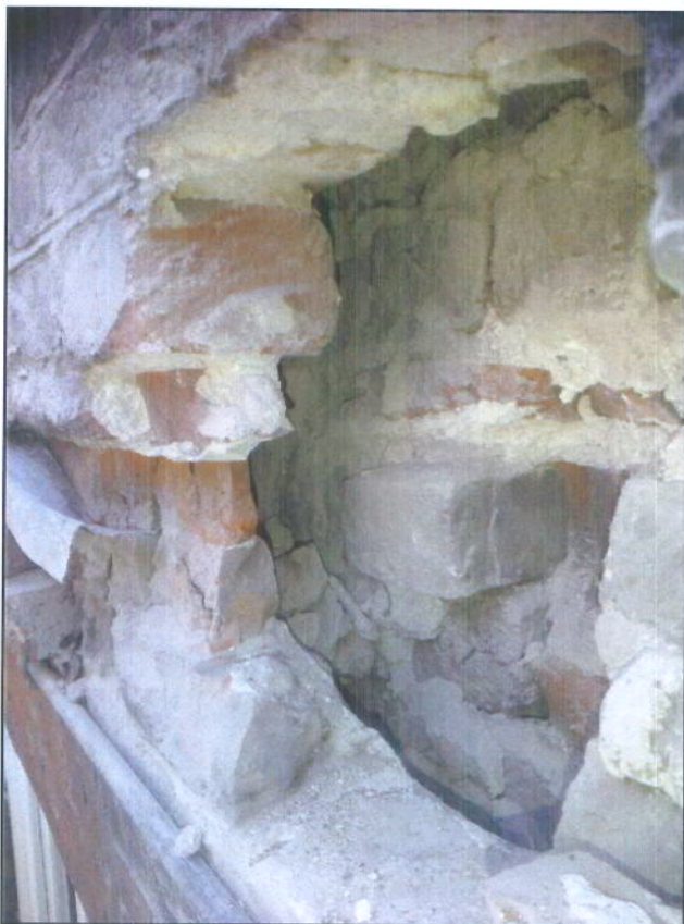
Photos 3-4. The gap created by separation of the external leaf.
