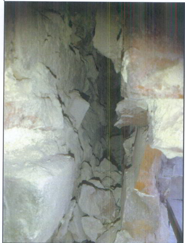
Photos 3-4. The gap created by separation of the external leaf.
