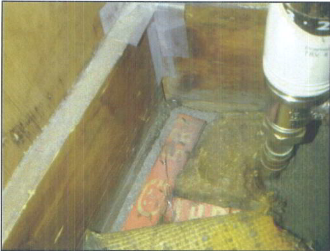
Photos 6-8. Cracks in the internal wood cladding (seal-taped due to draft and call air coming in through the cracks.)
