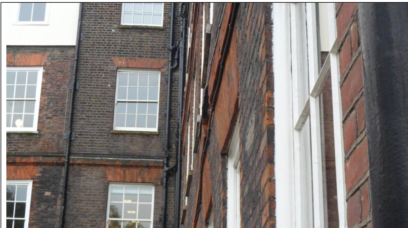
Photo 2: Bulging section of brickwork to front elevation
