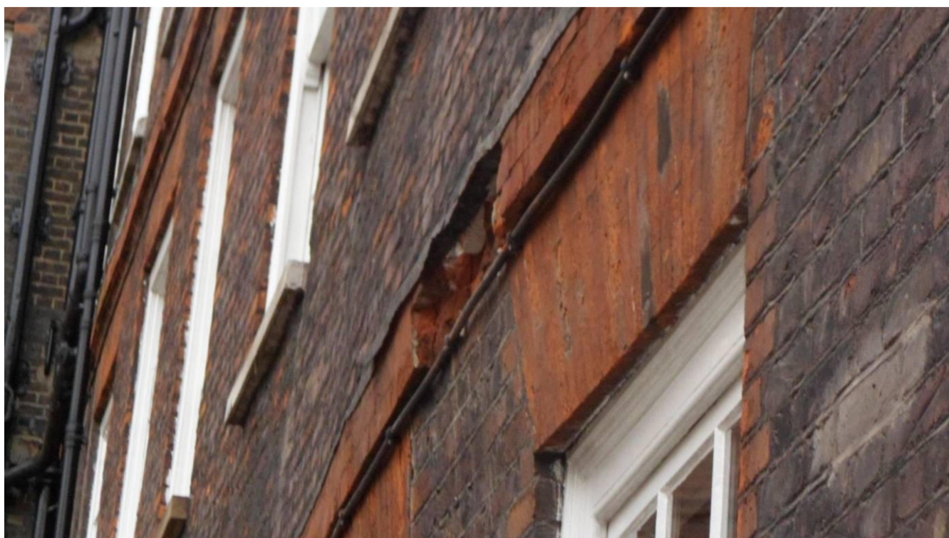
Photo 3: Closer view of bulging external brickwork wall to front elevation
