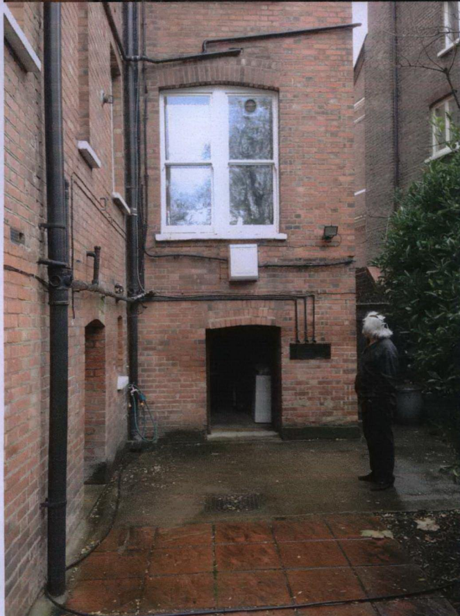
site of new balconies north rear elevation
