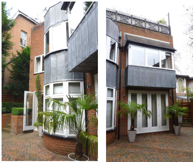
EXISTING REAR VIEWS
