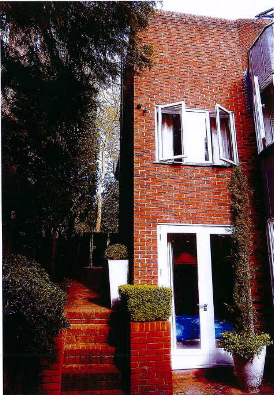
Photo 4. Rear (East) Elevation. Taken 10.05.10.
