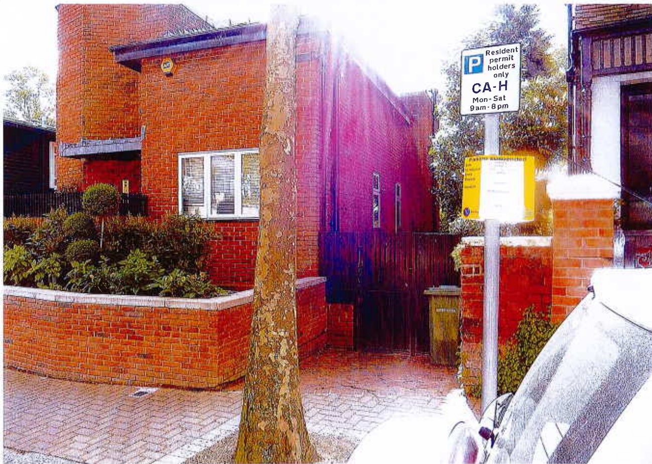
Photo 3. Front (West) Elevation. Taken 10.05.10.
