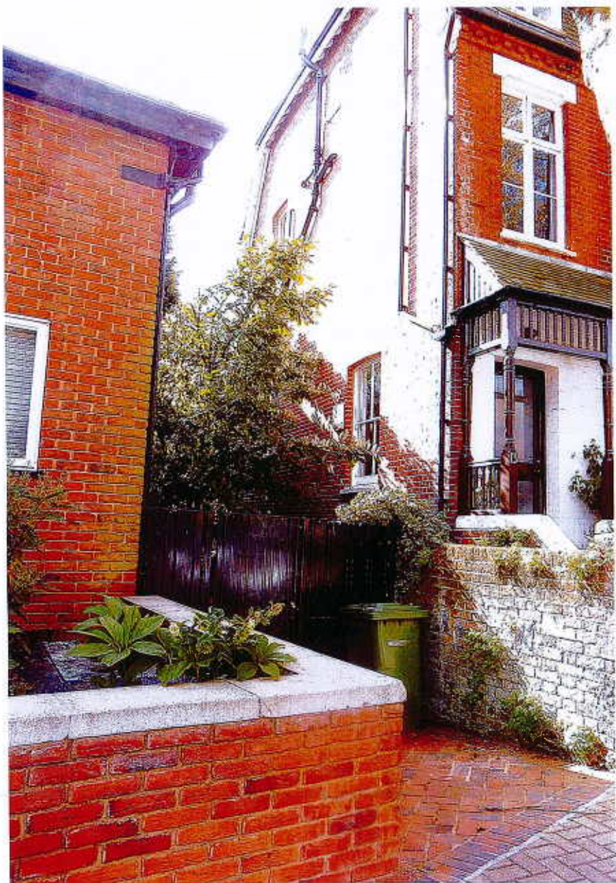
Photo 2. Front (West) Elevation. Taken 10.05.10
