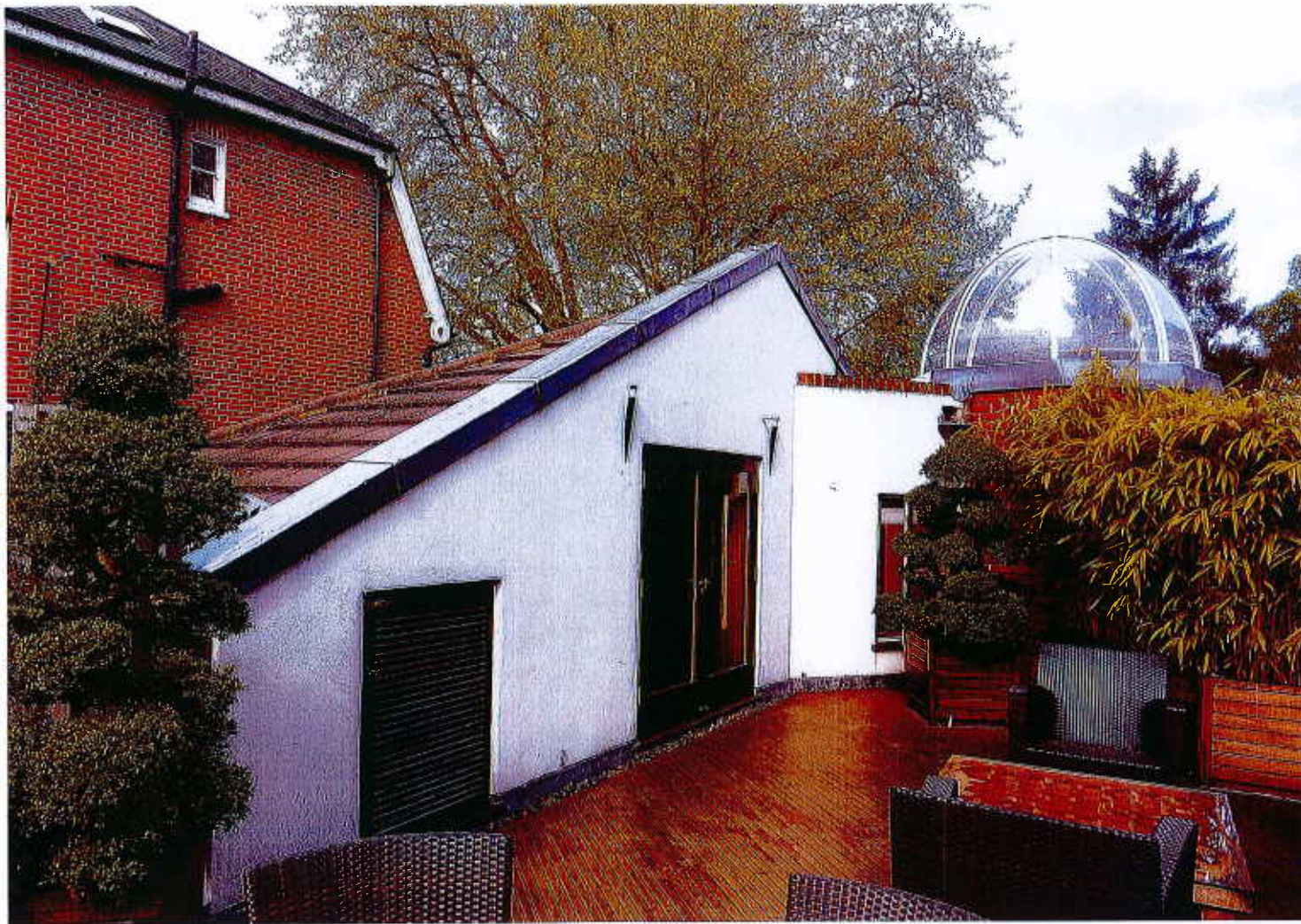
Photo 7. First floor roof terrace looking West. Taken 10.05.10.
