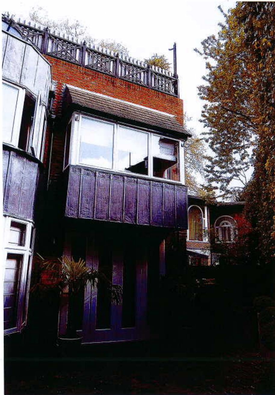
Photo 5. Rear (East) Elevation. Taken 10.05.10.
