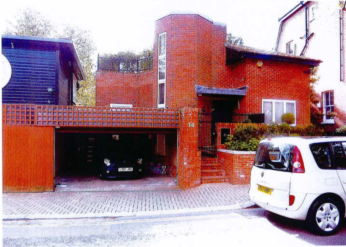
Photo 1. Front (West) Elevation. Taken 10.05.10.
