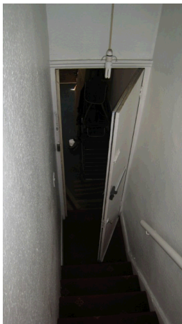
non-original handrails to be replaced with pigs ear handrail
