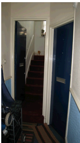
non-original handrails to be replaced with pigs ear handrail
