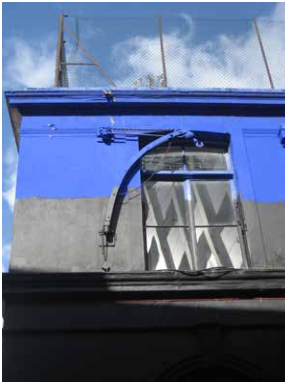
Fig. 3.12: Early metal crane on the first floor elevation.
