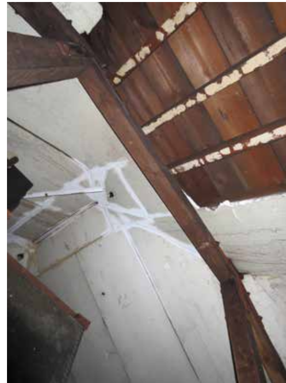
Fig. 3.14: Deteriorated condition of roof, showing timber trusses.
