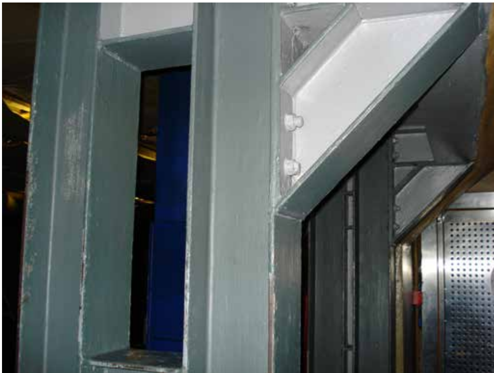
Fig. 3.20: Metal frame remedial support in No.16b West Central Street.
