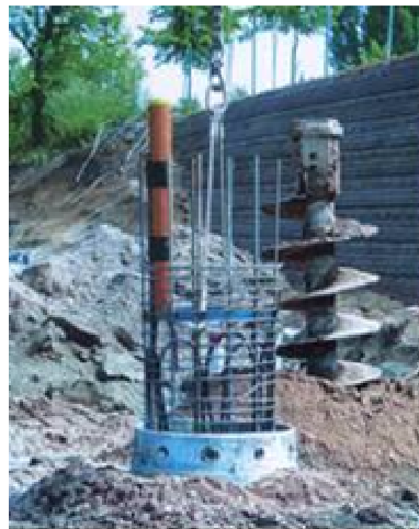
Ground level view – ground source energy pile
