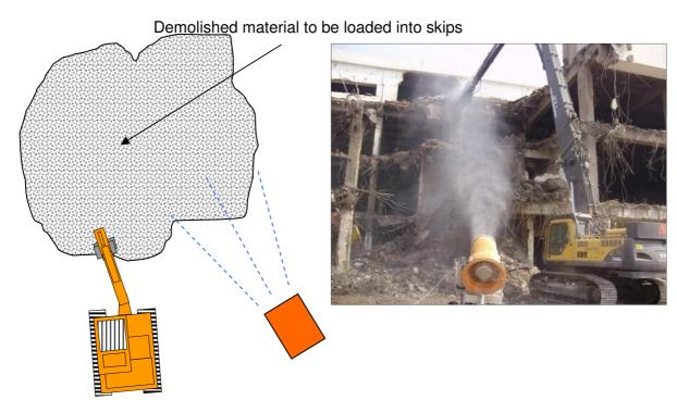
The Dust Boss would be located behind and to the rear of the demolition excavator, spraying a fine mist of water over the loading operation / dust source.
