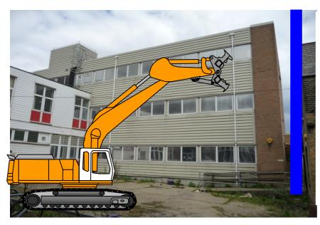
The construction of the units is concrete planks which sit on steel trusses; the excavator will demolish the building 1 bay at a time working in a top down sequence, ensuring the steel trusses are left intact; the brick work on the north elevation will be demolished by demolition operatives using hand held tools.
