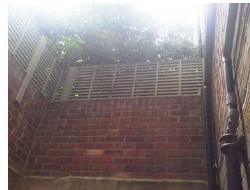
IMAGE OF EXISTING LIGHTWELL LOOKING TOWARDS TENANTS ABOVE FENCED TERRACE.
