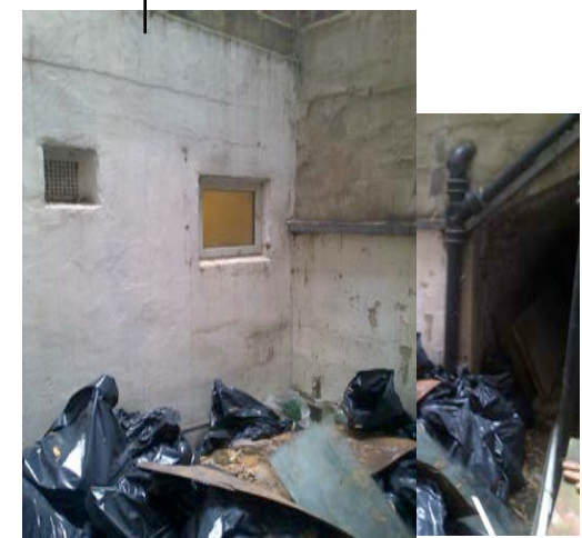
IMAGE OF EXISTING LIGHTWELL
