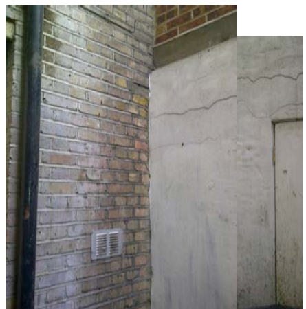
IMAGE OF EXISTING LIGHTWELL
