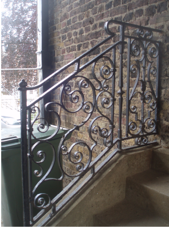
7. Original Metal Railings/ Central Extension - 1929
