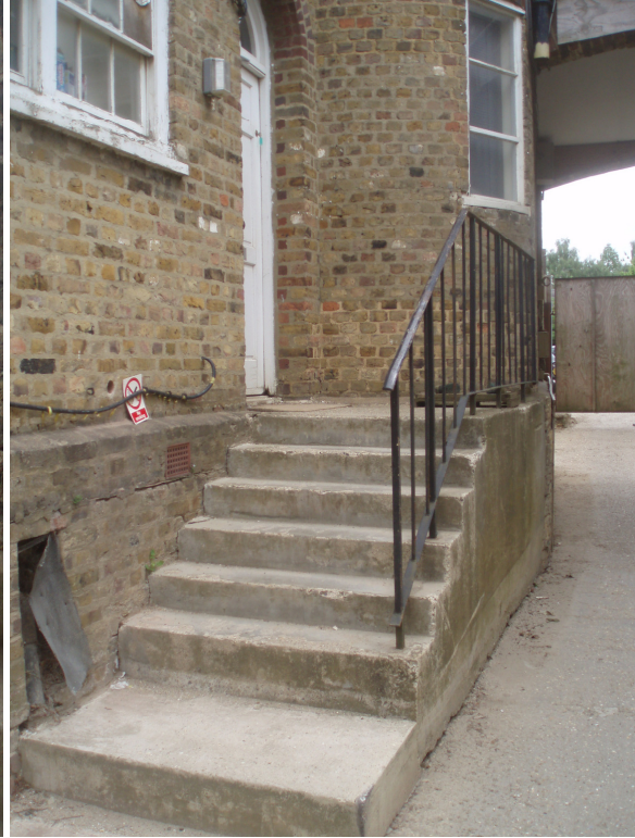
8. Modern Metal Railings – 1970's
