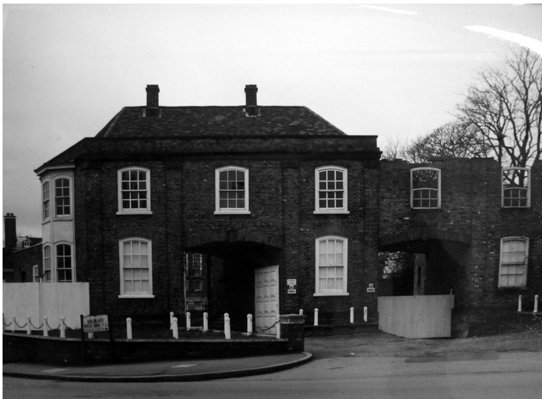
6. Existing Timber Gates - Archive 1970's
