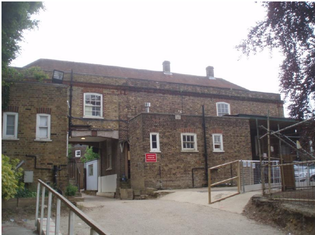
Figure 2: Rear of the Gatehouse
