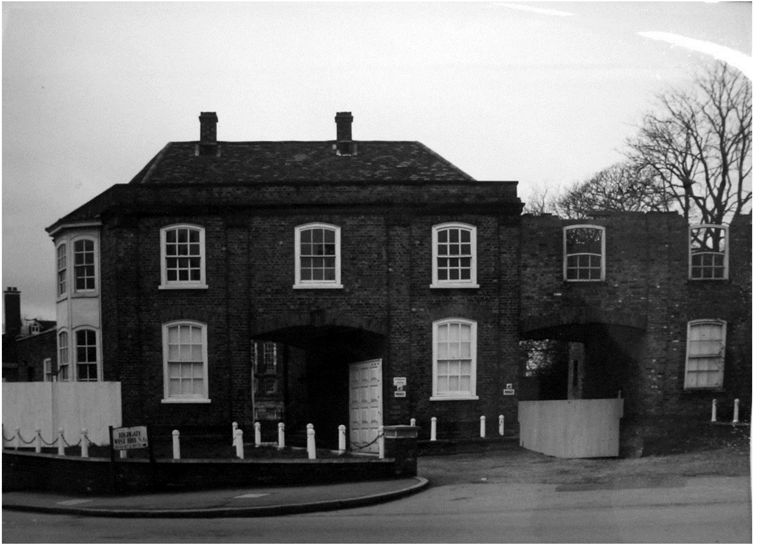
PROJECT H — GATEHOUSE PLANNING APPLICATION ARCHIVE PHOTOGRAPHS FROM 1970'S
