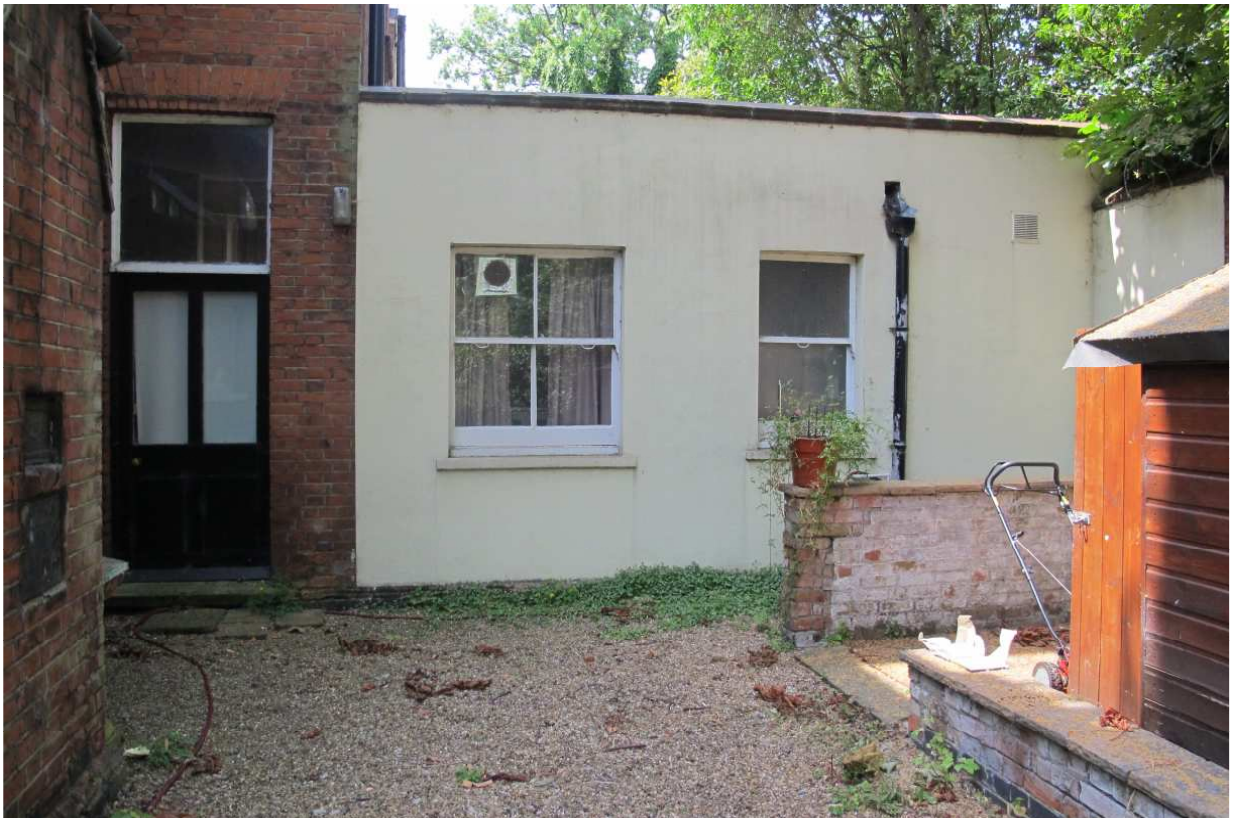
Photo 2. – Existing yard façade with door access.
