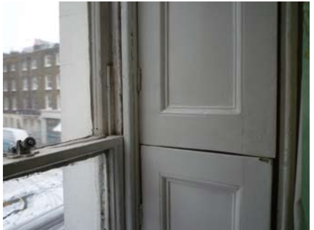
Fig 39 Timber shutter to front windows
