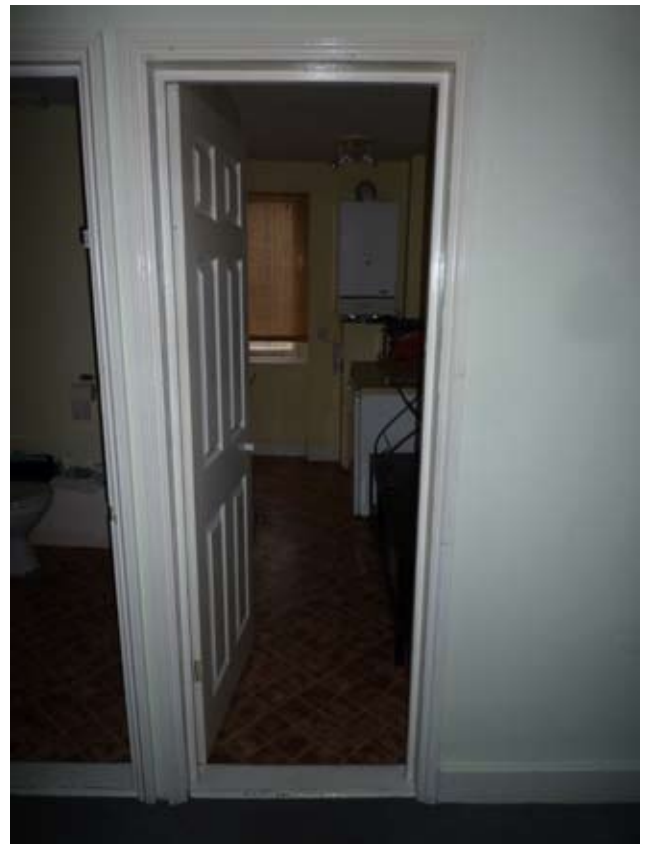
Fig 48 Openings in spine wall to kitchen and shower
