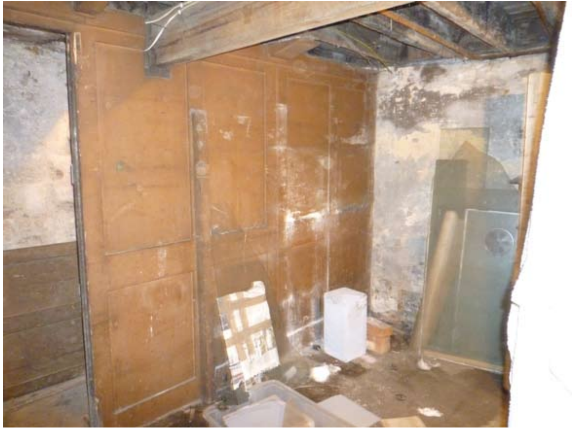
Fig 18 Timber partition within Basement below main building
