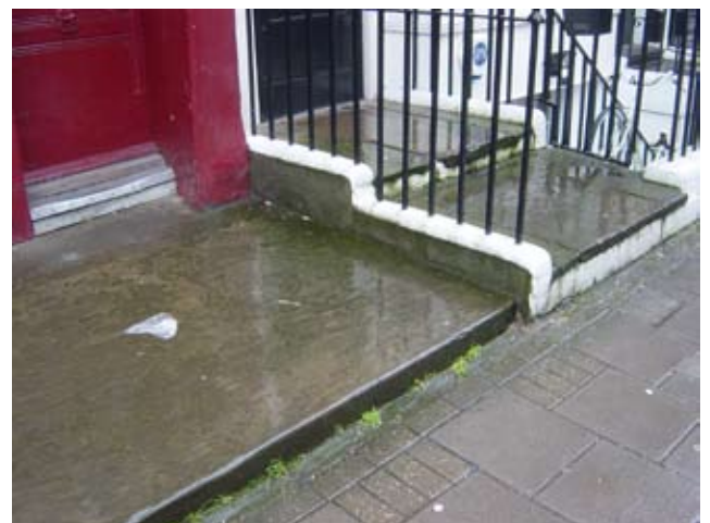
Fig 6 Concrete covering to front lightwell
