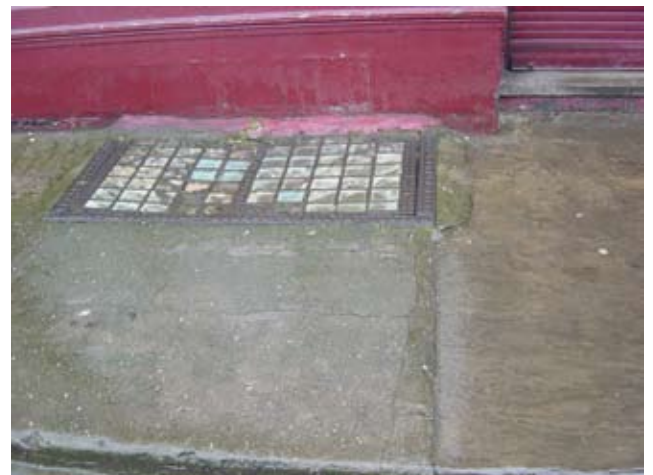
Fig 7 Pavement light to front lightwell
